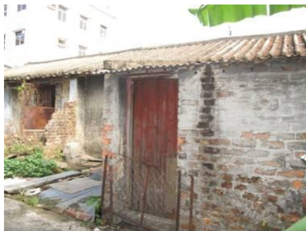
Photo 39 Village houses No. 77-80
