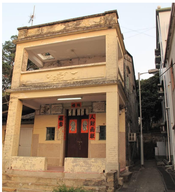
Photo 8 Frontview of village house No. 51
