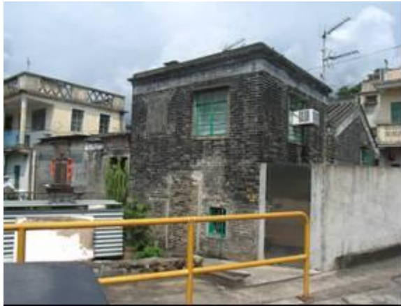
Photo 1 village houses No. 21-23
