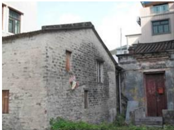
Photo 45 Sideview of building No. 18D
