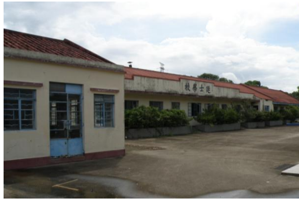
Photo 48 Ting Si School front view
