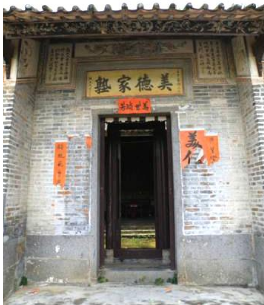
Photo 17 Façade of Mi Tak Study Hall
