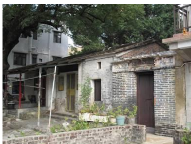
Photo 35 Village houses No. 93, 93A, 93B and 94
