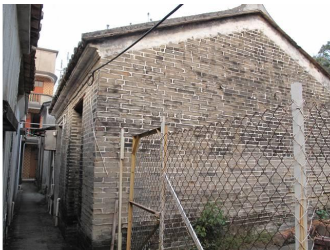
Photo 11 Sideview of village house No. 30C-31
