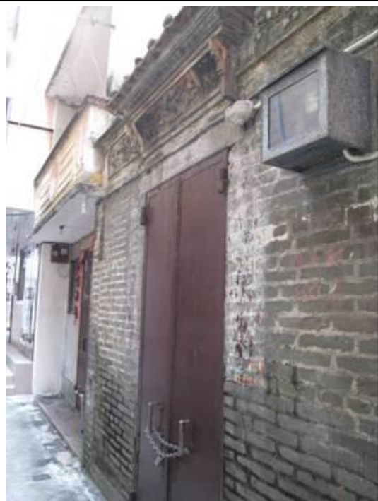
Photo 40 Frontview of village house No. 69
