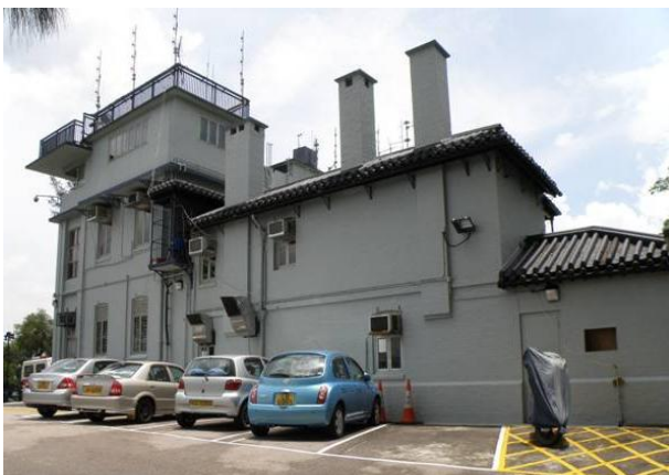
Photo 51 Sideview of LMC Police Station
