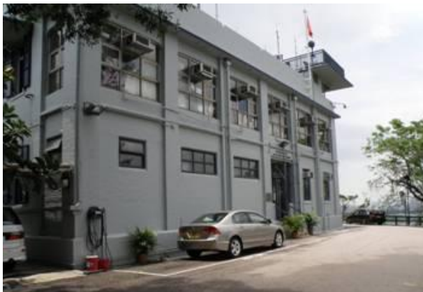
Photo 50 Sideview of LMC Police Station
