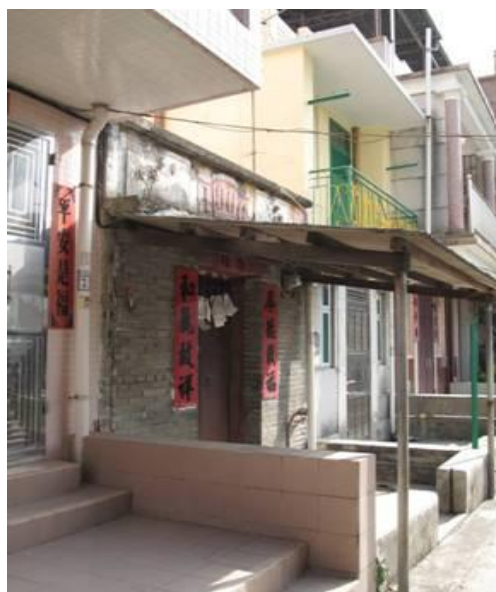
Photo 47 Frontview of village house No. 3
