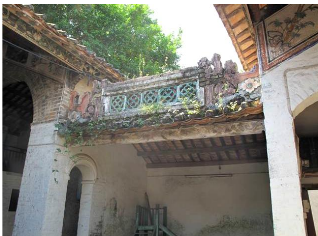
Photo 18 Interior walls and side chambers of Mi Tak Study Hall
