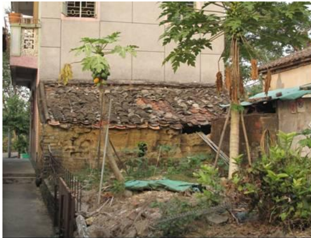
Photo 10 Sideview of the storage structure
