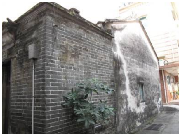
Photo 42 Sideview of the village house next to village house No. 64
