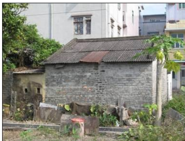
Photo 46 Sideview of unnumbered village house
