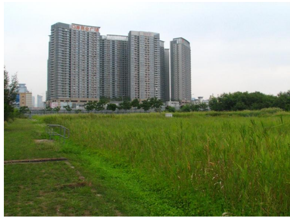
Plate 38. Clean-up reedbed at MTR LMC Station. A single cell of this facility will be temporarily lost during construction of Direct Link to LMC Station.
