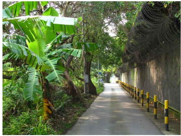
Plate 16. Ha Wan Tsuen Road, which will be upgraded to provide construction and operational phase access to LMC Loop. Adjacent habitats are currently rather disturbed.
