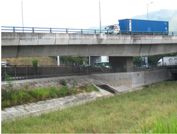
Plate 37. San Sham Road, linking San Tin Interchange with the boundary crossing point, alongside San Tin East Main Drainage Channel.
