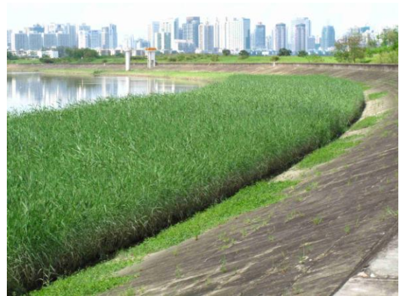
Plate 10. Shenzhen River. The channelized watercourse of the river is, in the section adjacent to LMC Loop, lined with a broad belt of reeds. These are cut at least annually.
