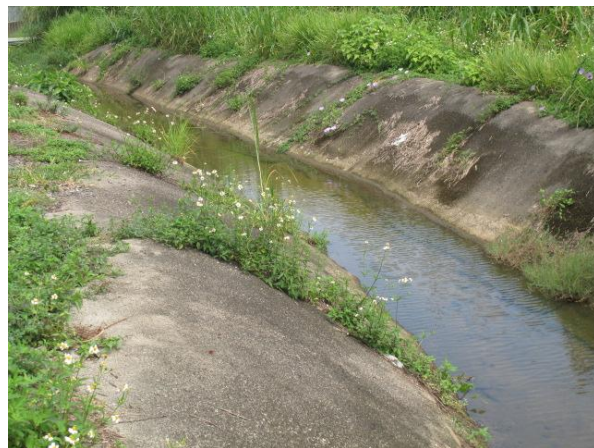
Plate 36. Ma Tso Lung Stream. Some sections of the stream are dominated by concrete banks, limiting ecological value.
