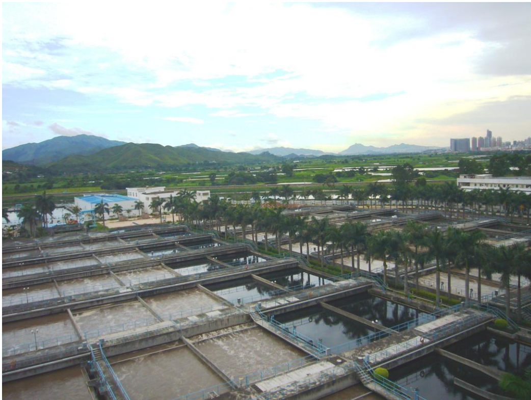
Photo 11 Residential buildings next to the aeration tanks
