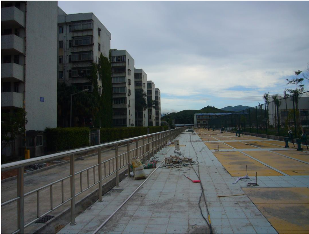
Photo 10 Residential buildings next to the sedimentation tanks
