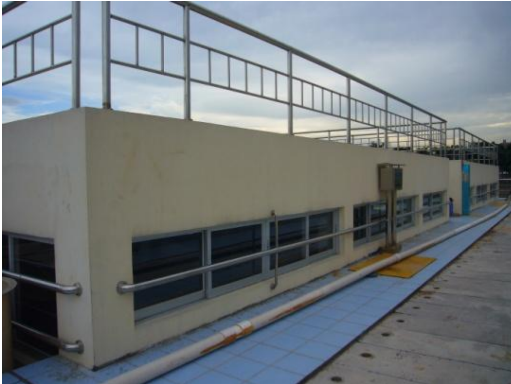
Photo 3 Biological treatment tanks are fully enclosed
