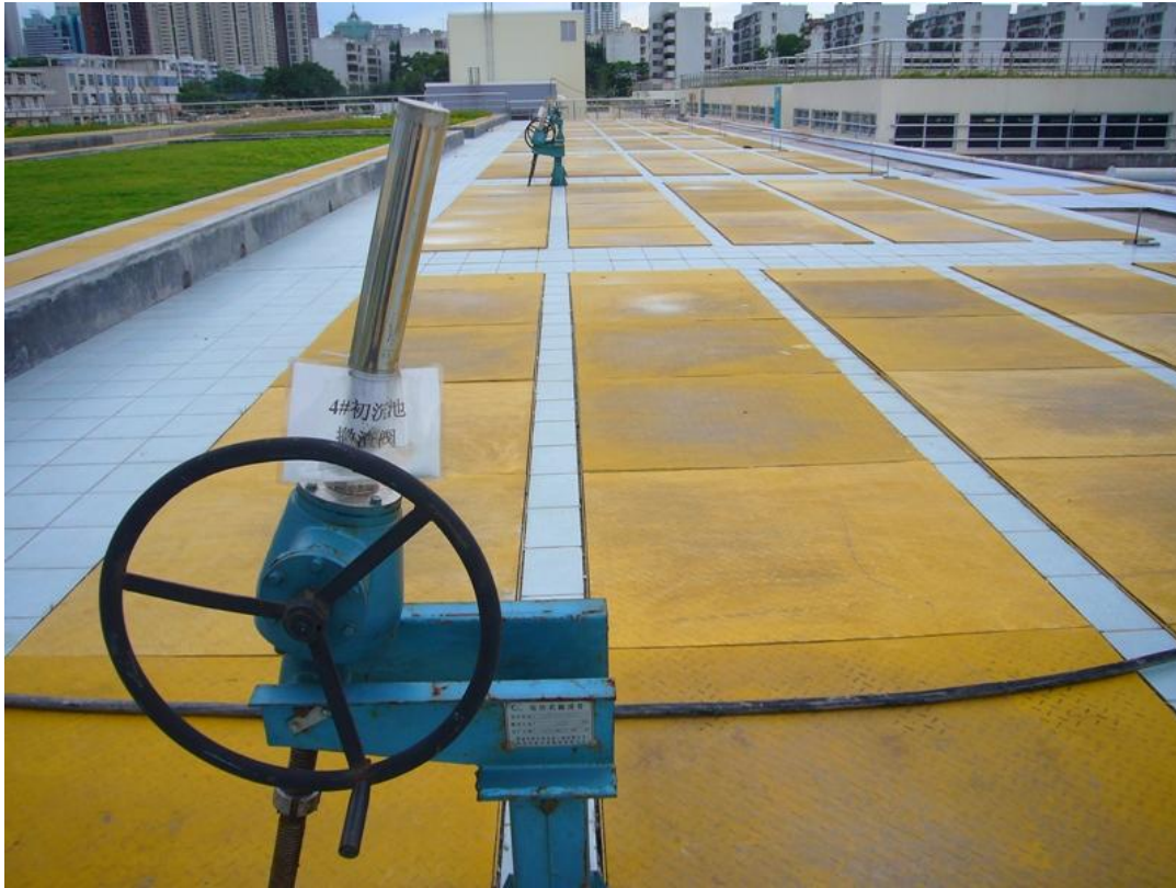
Photo 2 Primary sedimentation tank are fully enclosed.
