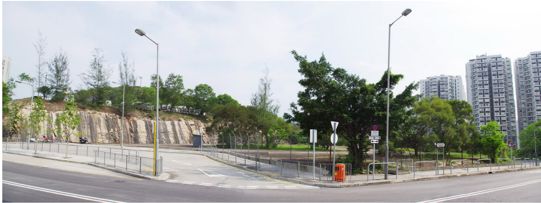
FROM LT-GIC2 Staff and Students of schools and Government facilities at Rehab Path
