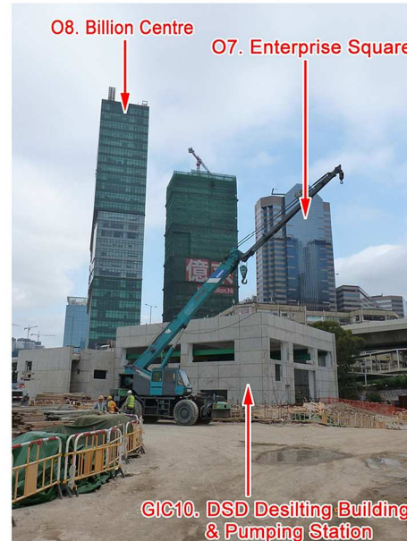
GIC10 – Jordan Valley Box Culvert: DSD Desilting Building & Pumping Station
