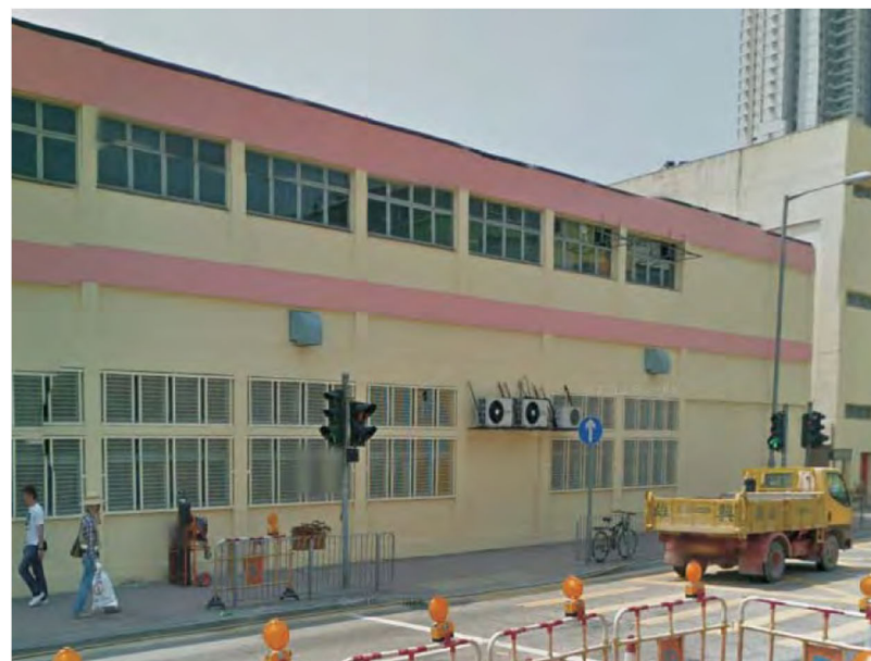
GIC1 – EMSD Workshops/Sewage Pumping Station & Electricity Substation
