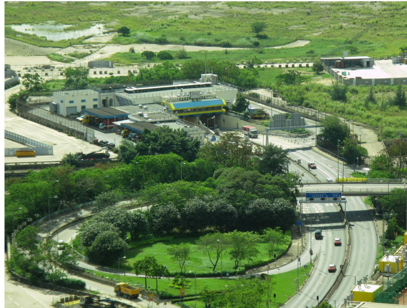
GIC4 – Tunnel Ventilation Shaft & Administration Building
