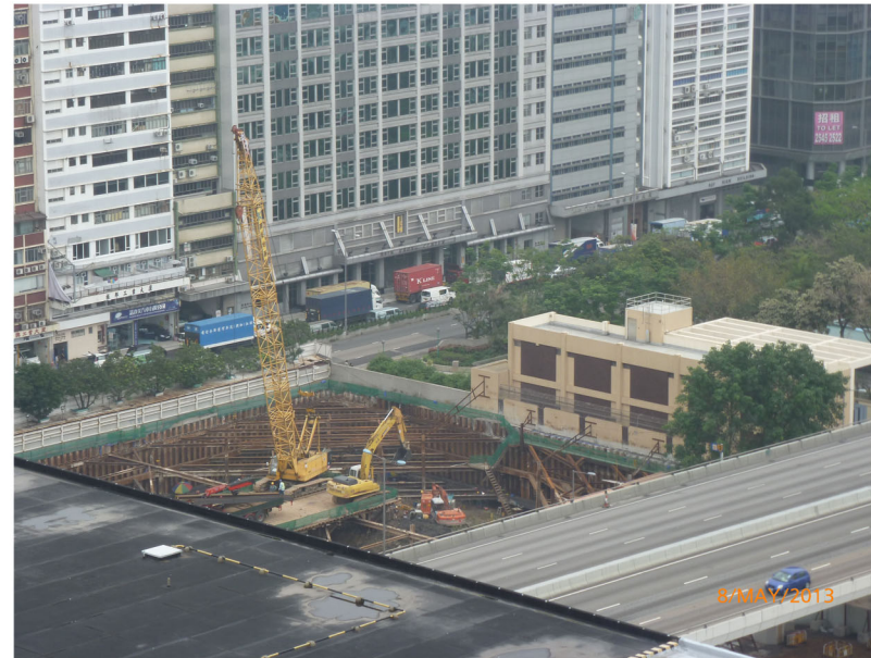
O20 – Soccer Pitch, Petrol, Car Park, Filling Station & vacant Sites/Proposed Cha Kwo Ling Promenade/Park
