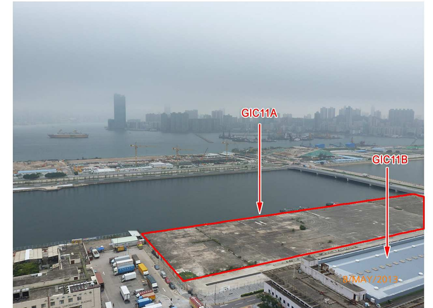
GIC11A – Hospital at former Kai Tak South Apron
