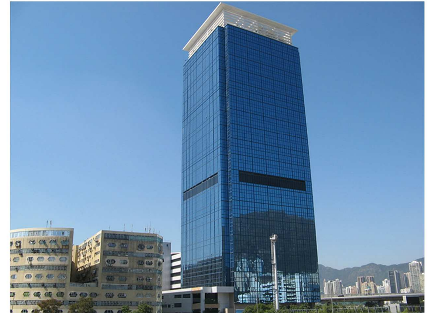
O3 – Skyline Tower, Kowloon Bay
