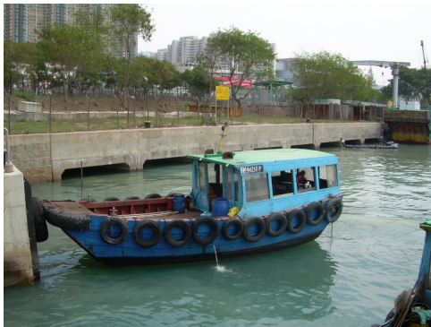
Drainage outfall near location F
