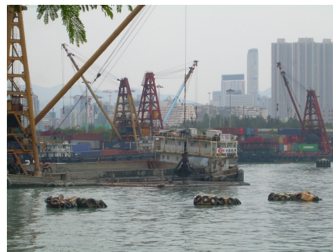
A barge was grabbing sediment from sea near location F
