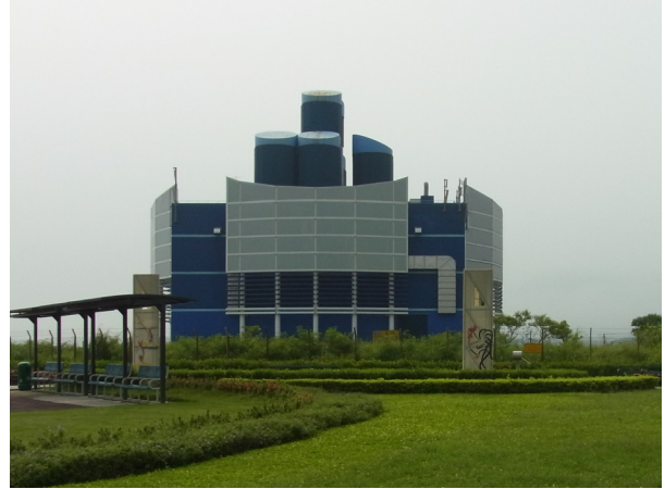
Photo 8 Ventilation building for the Western Harbour Crossing
