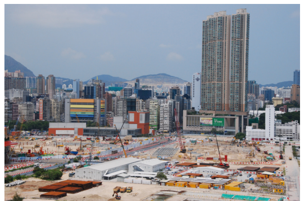
Photo 4 Temporary works area for XRL
