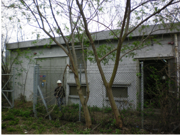
Photo 7 Seawater Pumping Station
