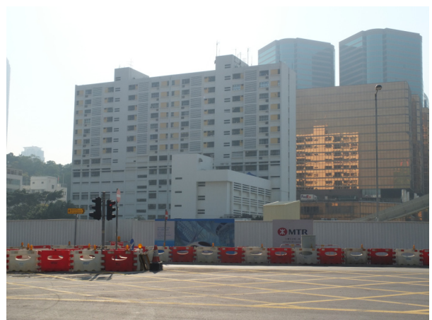
Photo 6 Tsim Sha Tsui Fire Station
