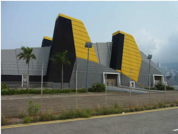
Photo 9 Ventilation buildings for the Airport Railway
