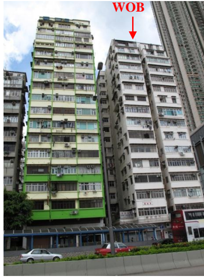
Wai On Building (WOB)
