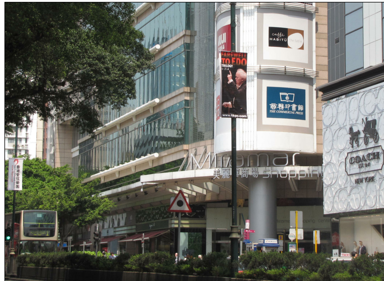
VSR 38 Miramar Arcade/ Tower and the Mira Hotel
