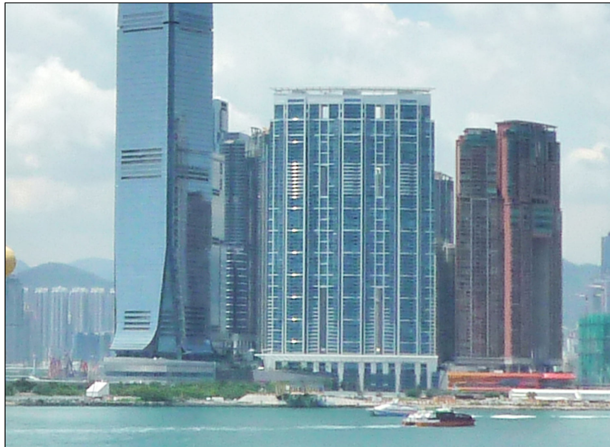
VSR 10 The Harbourside
