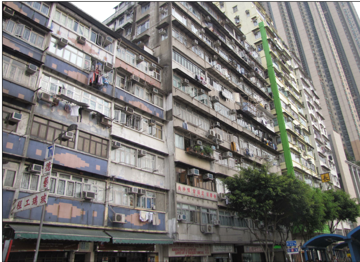
VSR 20 Wai On Building & Wai Hang Building
