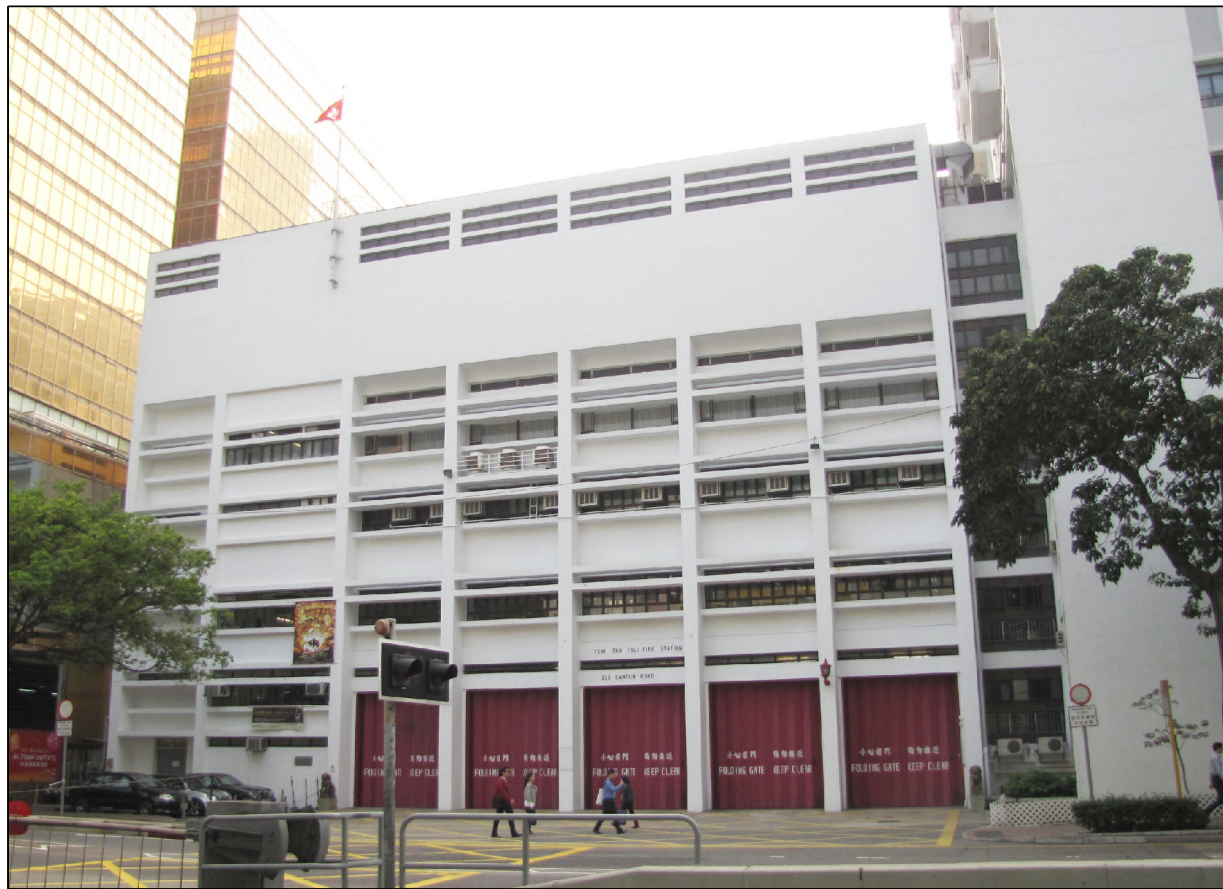
VSR 43 Tsim Sha Tsui Fire Station
