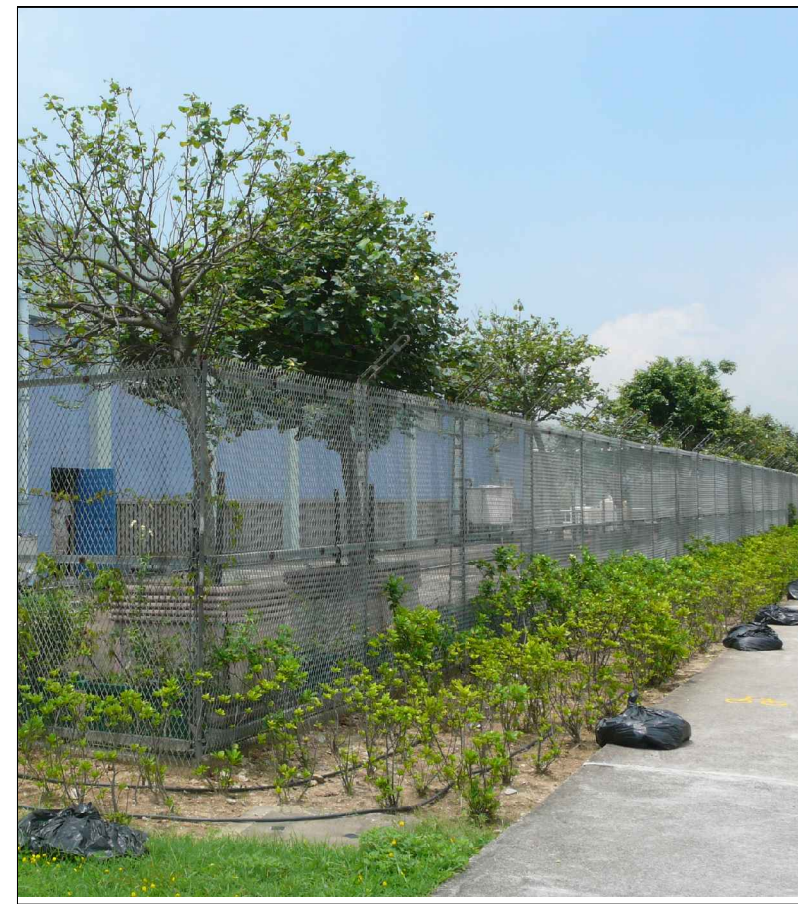
LR2.34 Amenity Planting within Salt Water Pumping Station Photo 1
