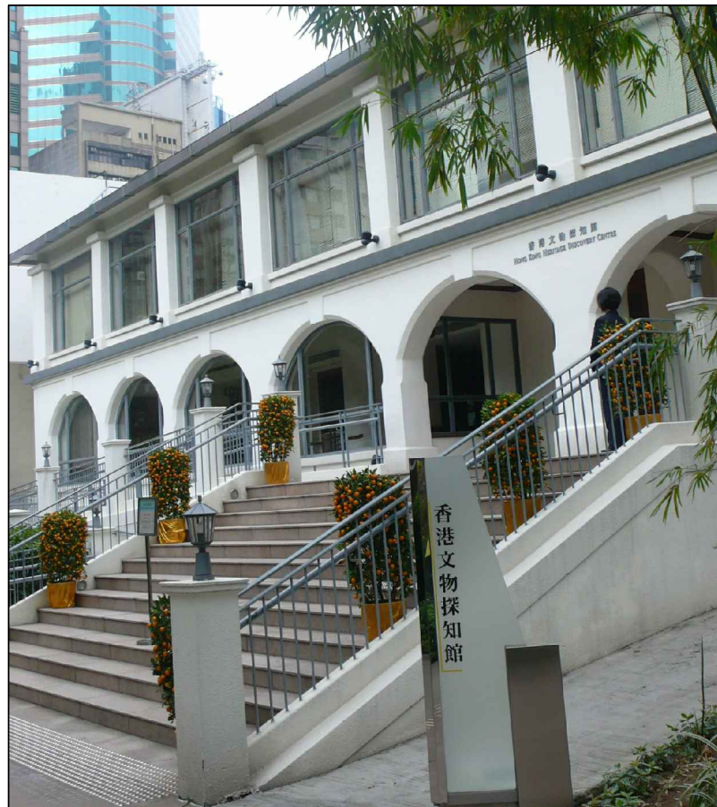
LR4.4 Built Heritage within Kowloon Park Photo 1 - Hong Kong Heritage Discovery Centre
