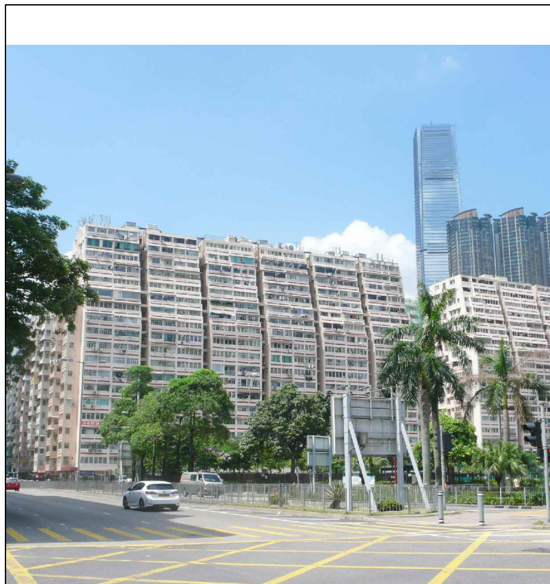
LR2.21 Roadside Trees along Ferry Street (near Yau Ma Tei Electric Substation) Photo 1
