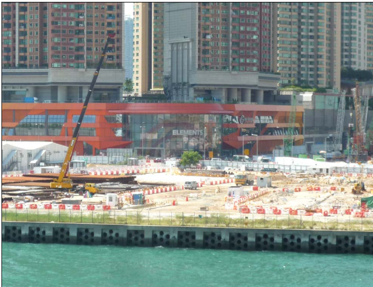
Photo VC03 (LCA02) West Kowloon Cultural District Construction Area
