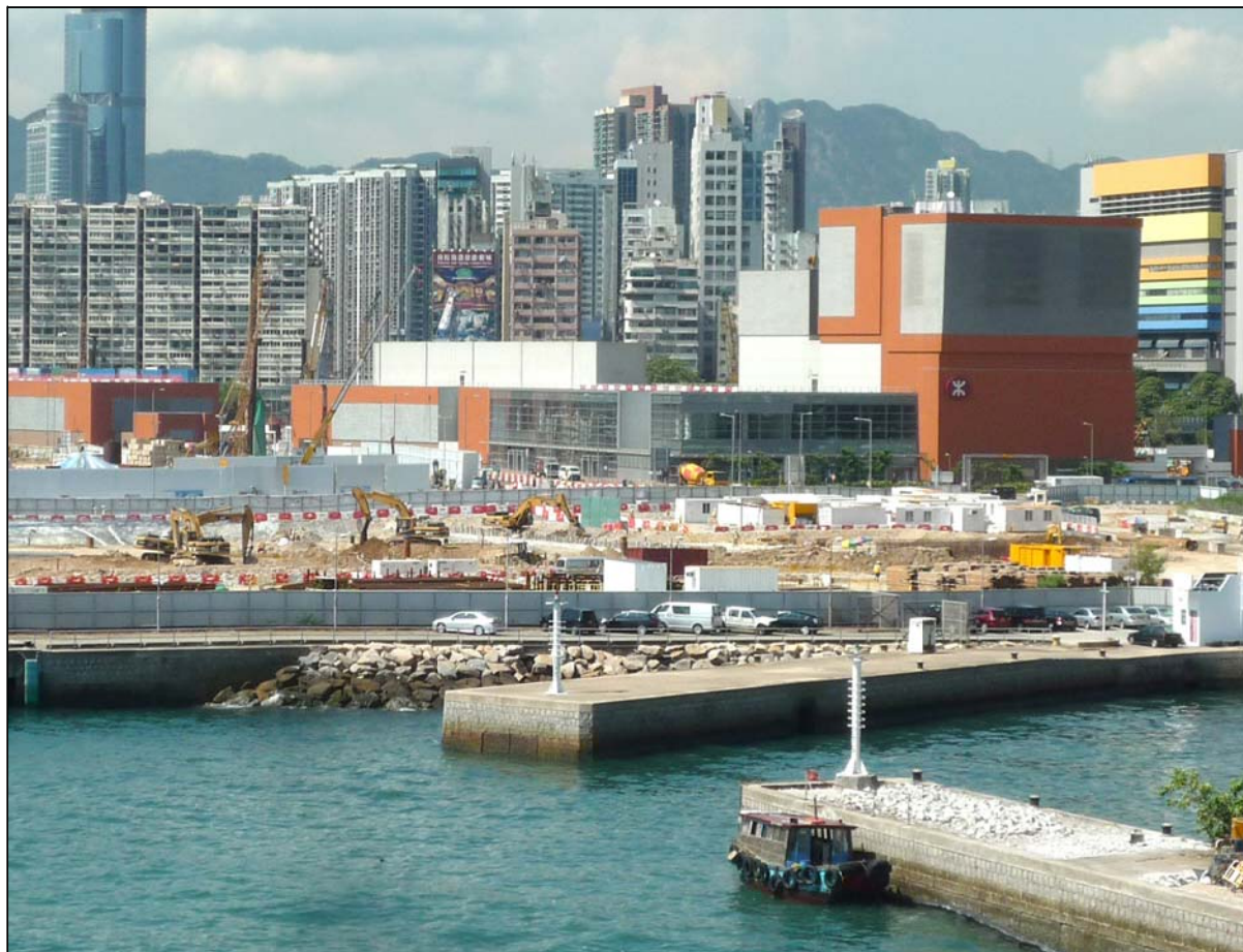
Photo VC04 (LCA02) West Kowloon Cultural District Construction Area
