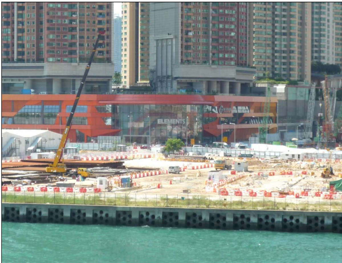
Photo VC03 (LCA02) West Kowloon Cultural District Construction Area
