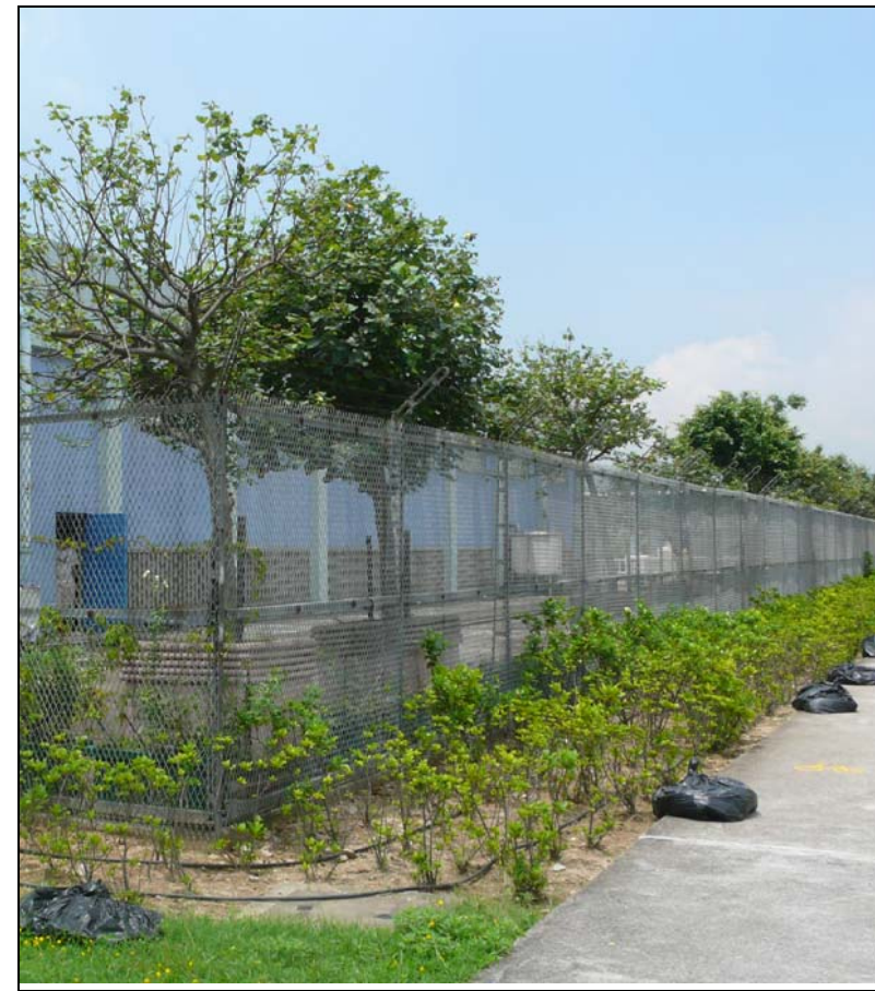
LR2.34 Amenity Planting within Salt Water Pumping Station Photo 1
