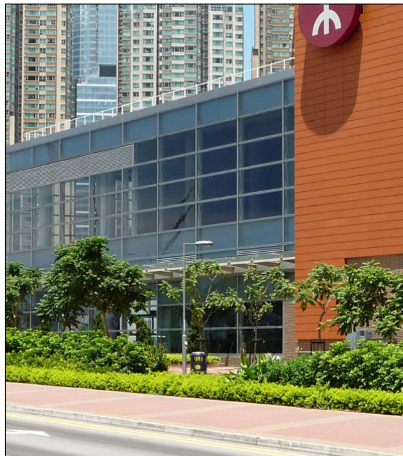
LR2.11 Roadside Plantation along Austin Road Photo 3
