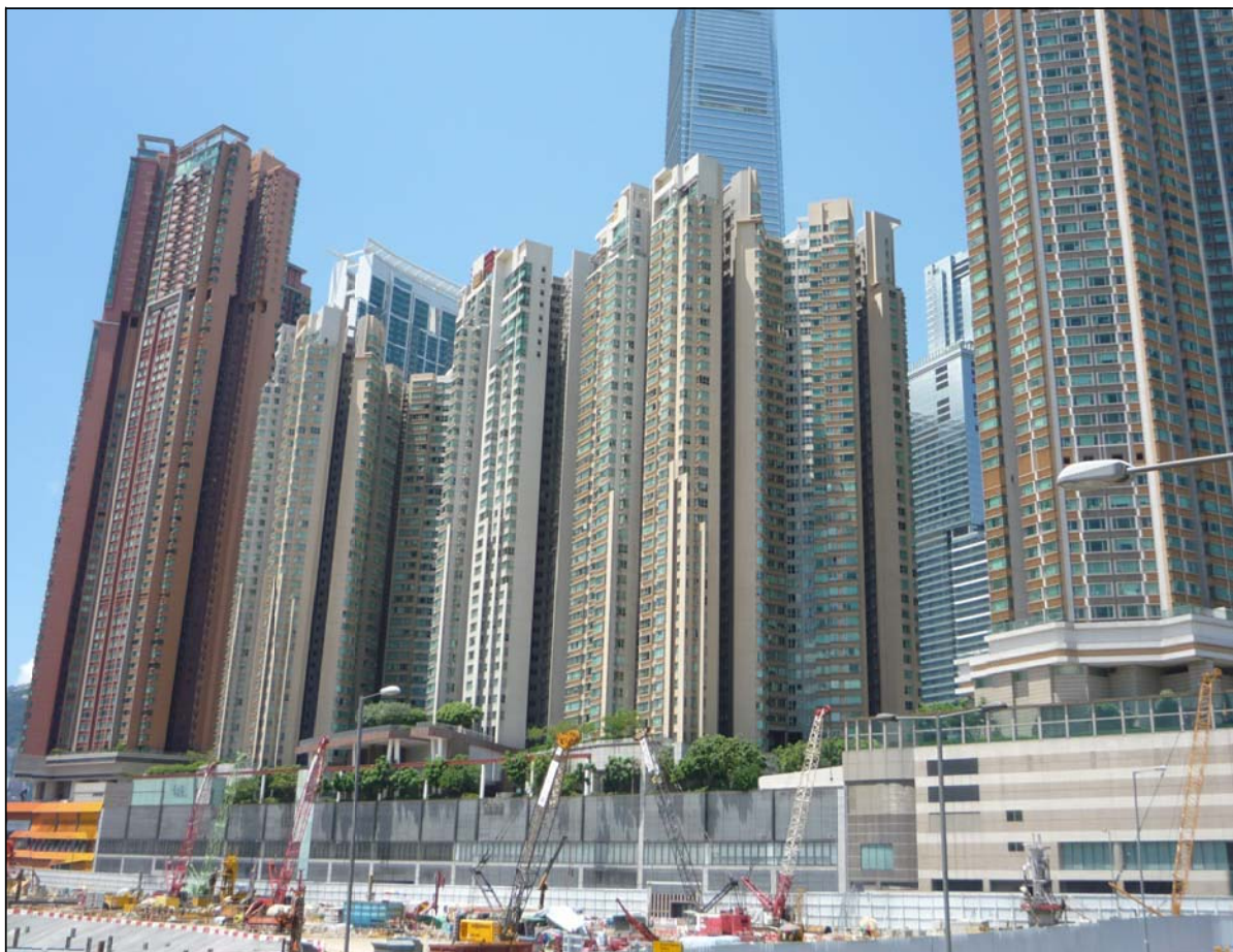
Photo VC18 (LCA09) Tsim Sha Tsui Late 20C/Early 21C Commercial/Residential Complex Landscape
