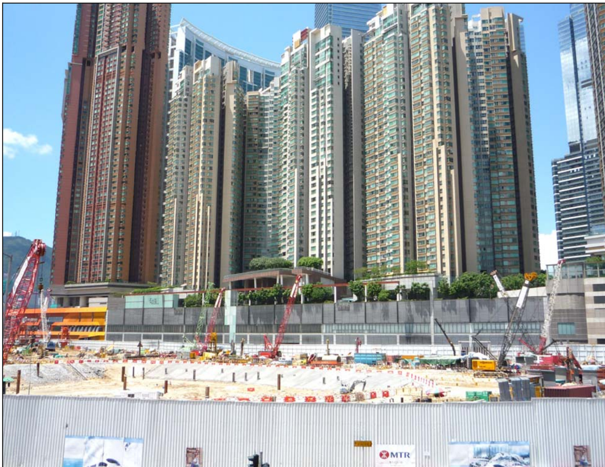
Photo VC20 (LCA10) Guangzhou-Shenzhen-Hong Kong Express Rail Link Terminus Construction Site & Austin Station
