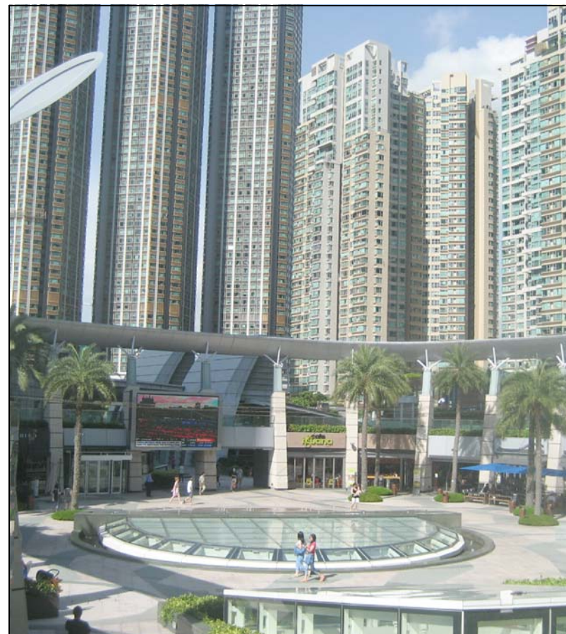
LR1.15 Public Open Space at the Kowloon Station Photo 1
