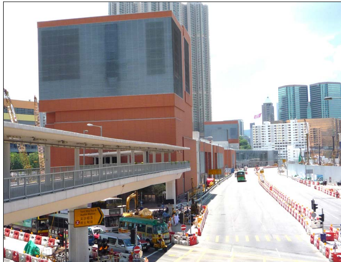
Photo VC19 (LCA10) Guangzhou-Shenzhen-Hong Kong Express Rail Link Terminus Construction Site & Austin Station
