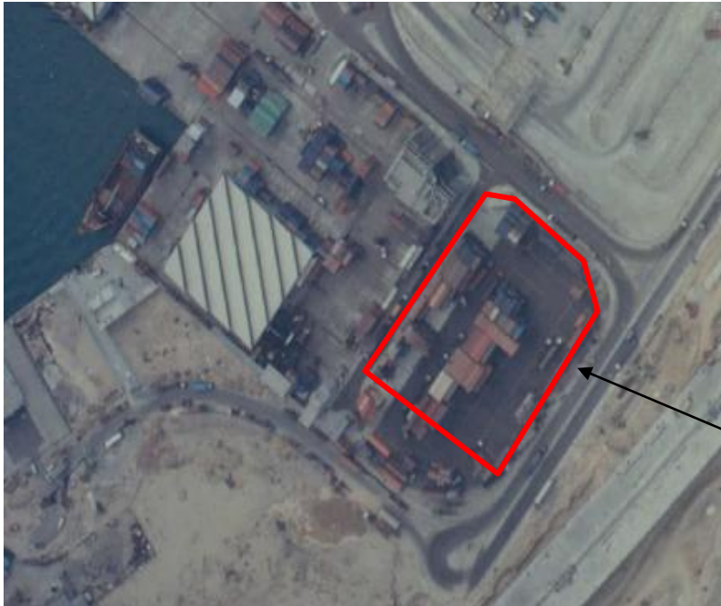
Figure 3 Project Site in Year 1995 (Photo No. CN11293)
