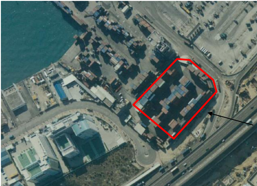
Figure 4 Project Site in Year 2001 (Photo No. CN30189)
