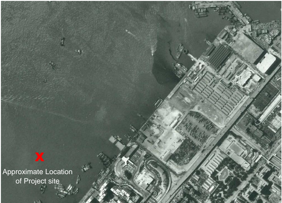
Figure 1 Coastal Area before Reclamation in Year 1991 (Photo No. A28859)
