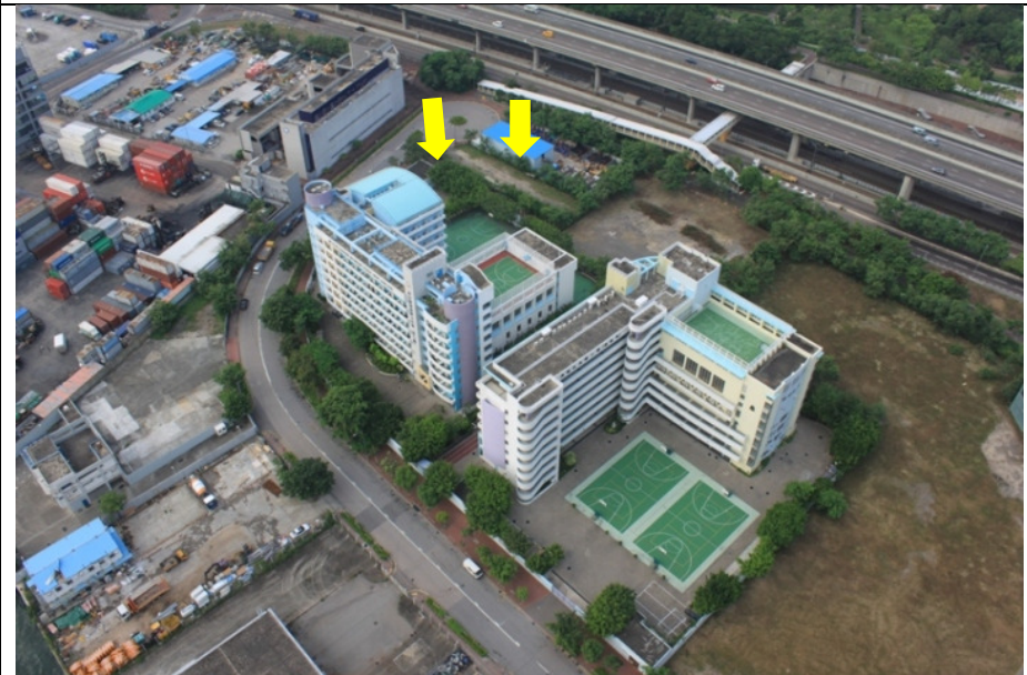
LR 5-5 In between the vacant land to the northeastern of Sir Ellis Kadoorie Secondary School (West Kowloon)
