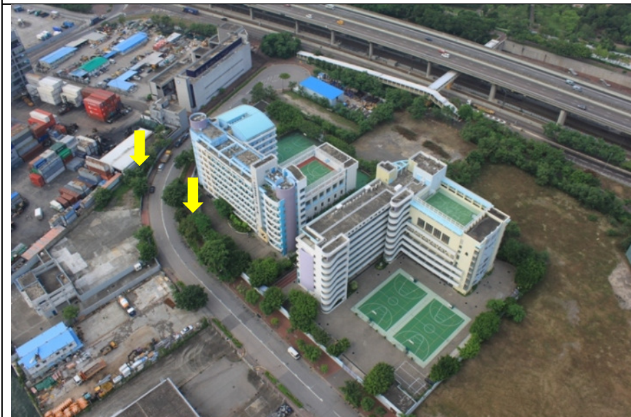
LR 2-3 Along Hoi Fan Road
