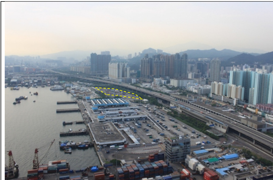
LR 4-1 To the west of Wholesale Fish Market along Lin Cheung Road, bounded by Lin Cheung Road and the marine frontage
