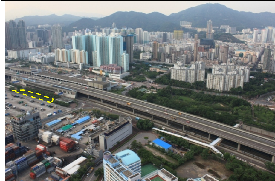
LR 5-2 Behind Nam Cheong Station Exit, along Wholesale Market Street, to the northwest of the Site
