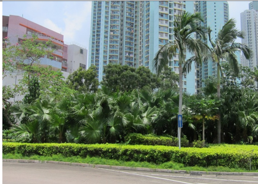
LR 6-10 To the southwest of Sewage Screening Plant of DSD amid Fu Cheong Estate and Nam Cheong Estate
