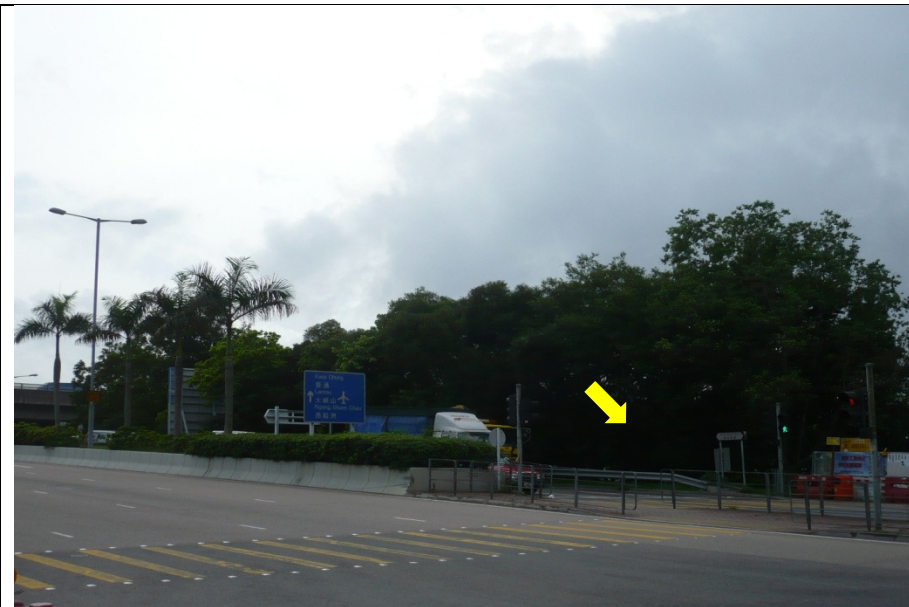
LR 5-7 At the slope next to bus terminal at Tonkit Street West
