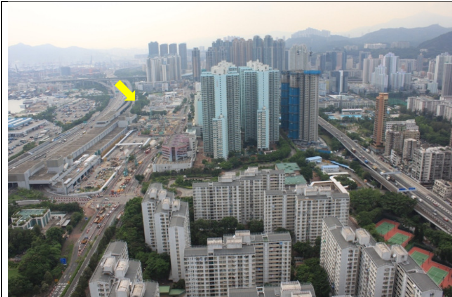
LR 2-9 Along Tonkin Street West
