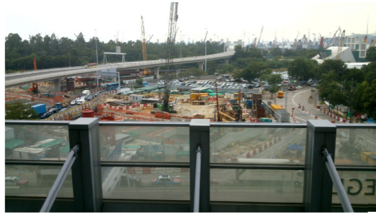
LR1.1 Roadside Amenity Planting - West Kowloon Highway
