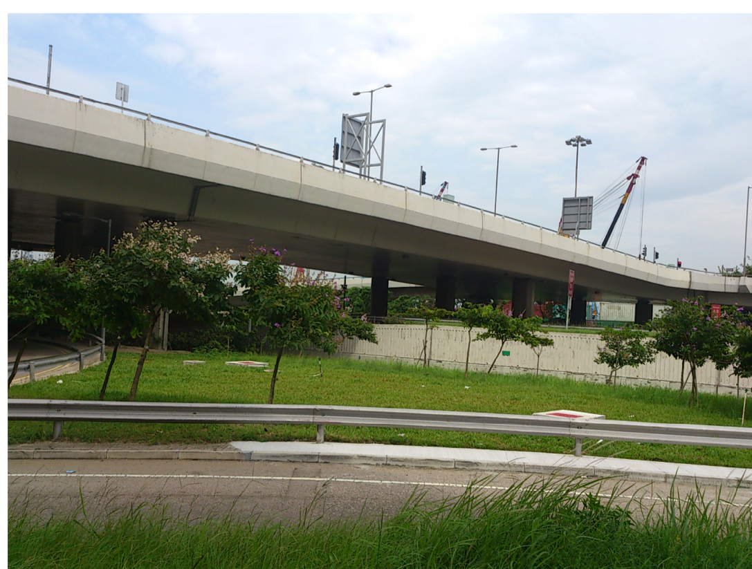
VSR13 - View from CLP Power Centenary Substation at To Wah Road
