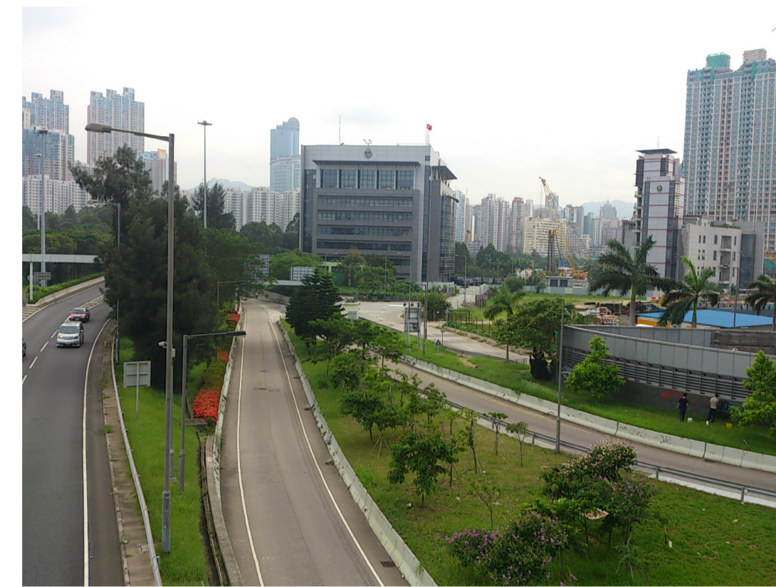
VSR8 - View of Civil and Service Headquarter
