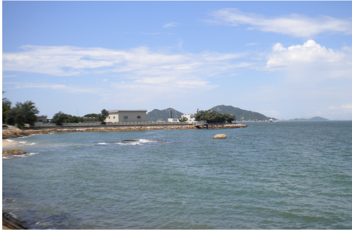
Existing View of the Cheung Chau STW
