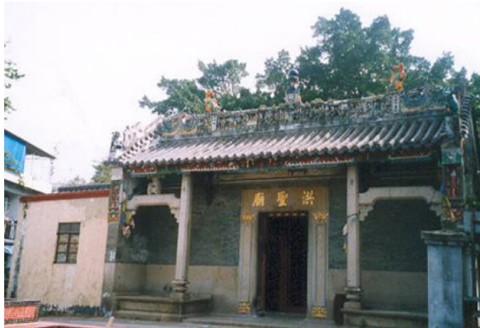
Exterior Façade of the Hung Shing Temple
