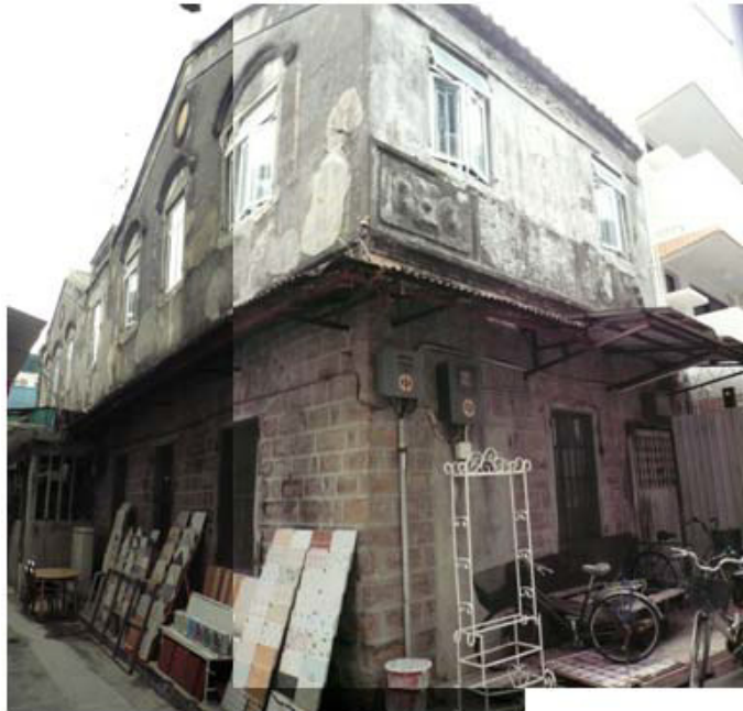
Rear and side elevation of Goon Sor
