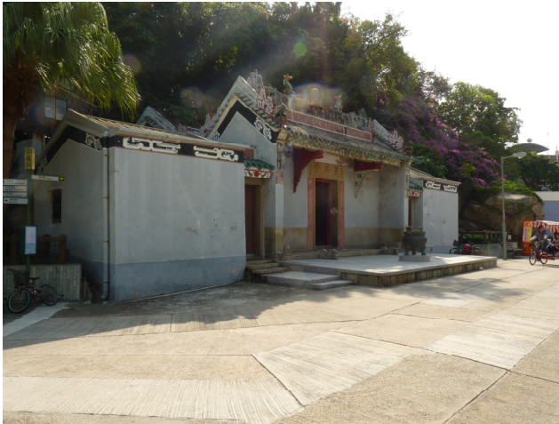
View of the Tin Hau Temple Façade
