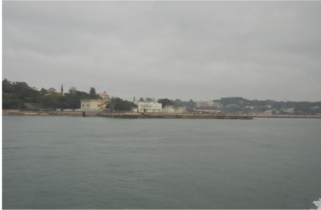
Existing View of the Cheung Chau STW
