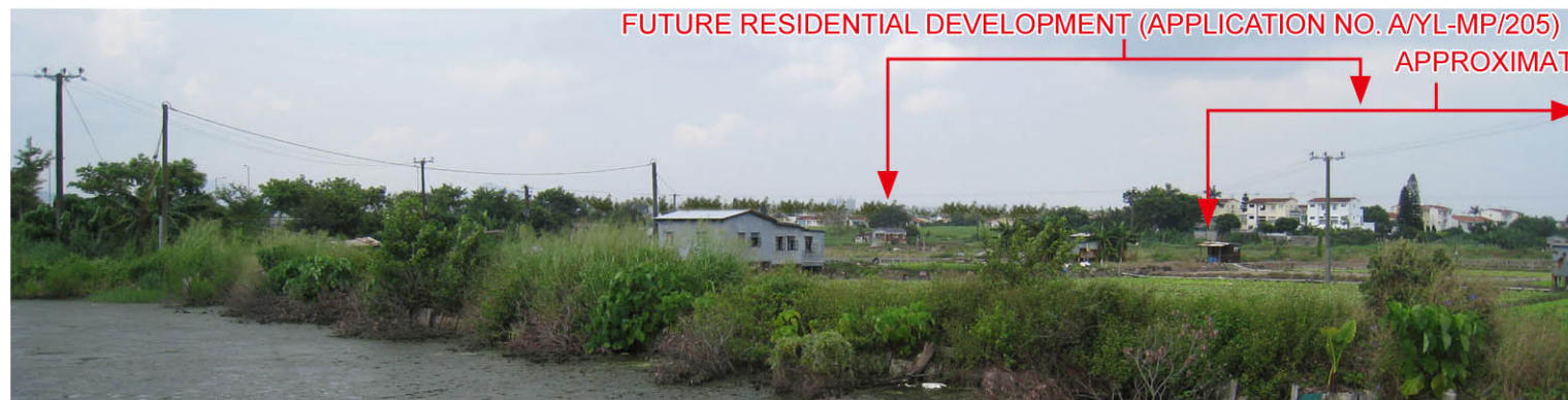
V9 – VIEW FROM YAU MEI SAN TSUEN (VSR NO. R3) - YEAR 10 WITH MITIGATION
