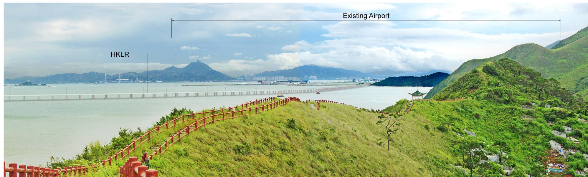
Planned Baseline Conditions in 2016 Before Commencement of the 3RS (with Committed and Approved Projects: HKBCF, HKLR, the Southern Connection of TM-CLKL, Residential/Commercial Development at Tung Chung (Area 55A), Residential Development at Tung Chung (Area 55B) and Residential Development at Tung Chung (Area 56))
