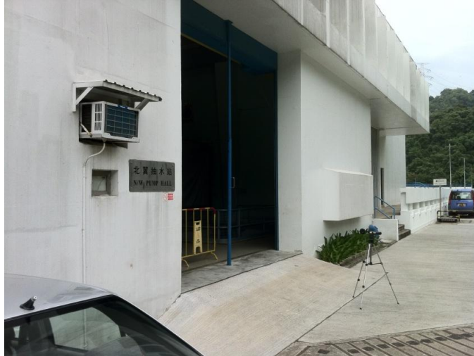
Fig. 4. North Pump Hall
