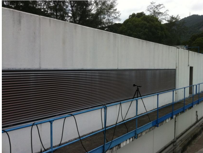
Fig. 2. Sludge Treatment House Ventilation
