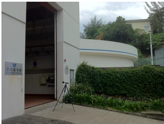
Fig. 3. Sludge Treatment House Front Opening
