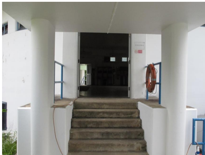
Fig. 5. Acceleration Tank Control Room
