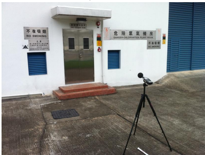
Fig. 8. Chlorine House (Ventilation)
