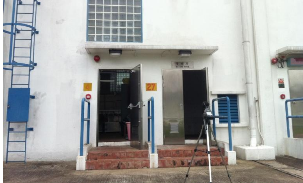
Fig. 9. Chlorine House (Battery House)
