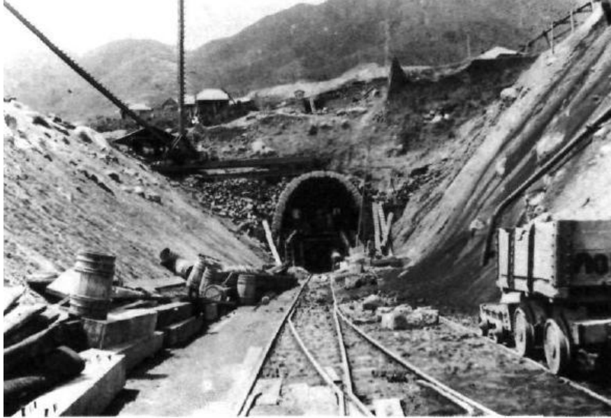
EX KCR Beacon Hill Tunnel Portal under construction, ca.1908.
