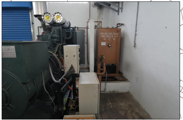
GENERATOR HOUSE (AREA H ~18m 2 )
