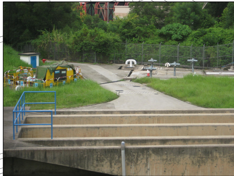
LAWN BESIDE ACCESS ROAD TO WASHWATER RECOVERY TANKS (THE SCENE OF CRANE LORRY OVERTURN INCIDENT) (AREA J)
