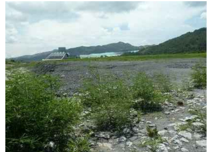
B - SURFACE OF ASH LAGOON FILLED WITH PFA TO 10.5 mPD
