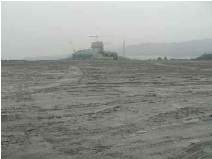
B - ABOUT 2/3 SURFACE OF ASH LAGOON FILLED WITH PFA
