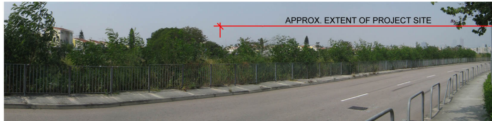
VIEW FROM VSR O3 CHUK YUEN FLOOD WATER PUMPING STATION - DAY 1 WITHOUT MITIGATION (VIEW POINT 15)
