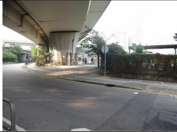
Photo 1: Entrance of Public Works Regional Laboratory Under Tsuen Wan Road
