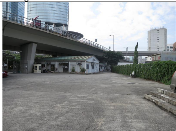
Photo 14: Public Works Regional Laboratory under Tsuen Wan Road
