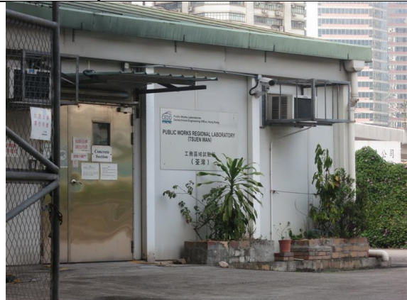
Photo 3: Front Side of Public Works Regional Laboratory
