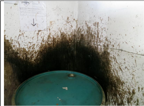
Photo 9: Wall in Storage Room for Chemical Waste
