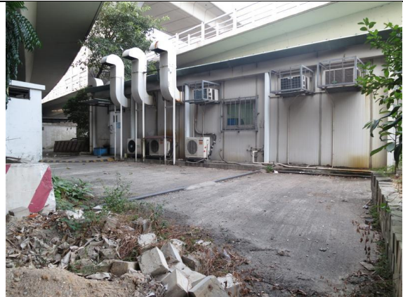
Photo 4: Back Side of Public Works Regional Laboratory
