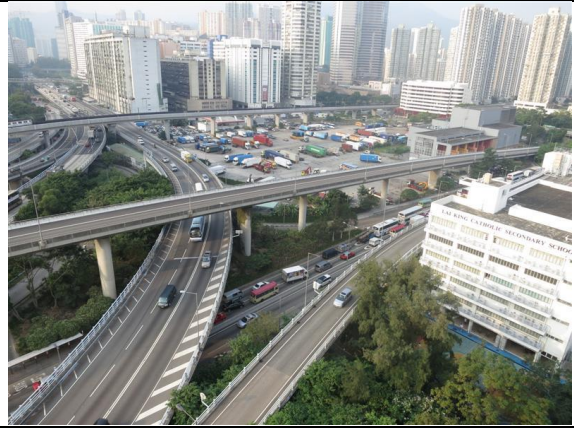
Photo 2: Aerial View of Tsuen Wan Road
