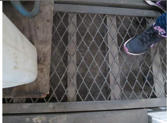
Photo 8: Mesh Floor of the Storage Room for Chemical Waste
