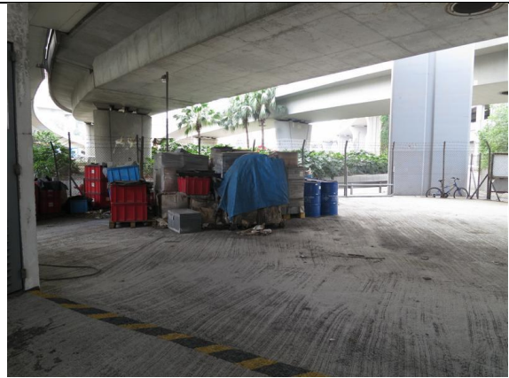
Photo 10: Outdoor Storage Area
