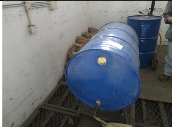
Photo 7: Tank for Fresh Methylene Chloride
