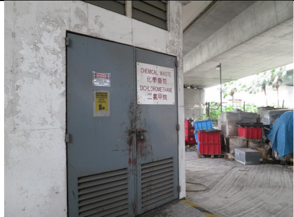
Photo 6: Storage Room for Chemical Waste
