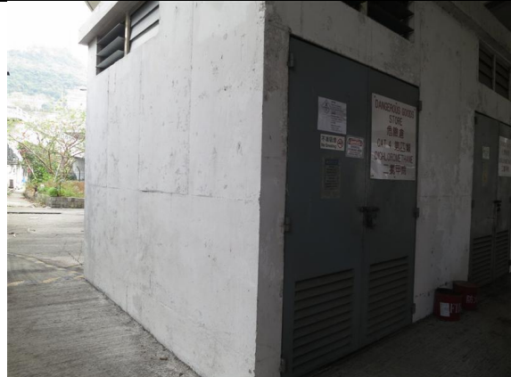
Photo 5: Dangerous Goods Store
