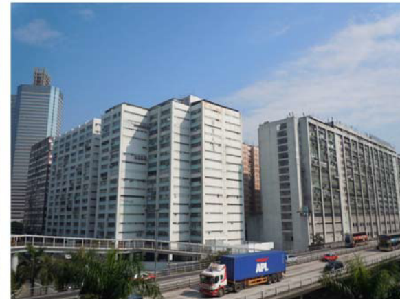
LCA4 Industrial & Open Storage Area along Tsuen Wan Road
