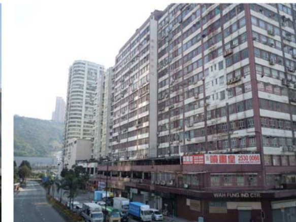
■ O2 Workers at Kwai Chung Industrial Area
