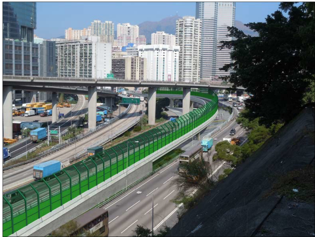
CASE 3 - PROPOSED FLYOVER FROM KWAI TSING INTERCHANGE UP-RAMP TO KWAI CHUNG ROAD
