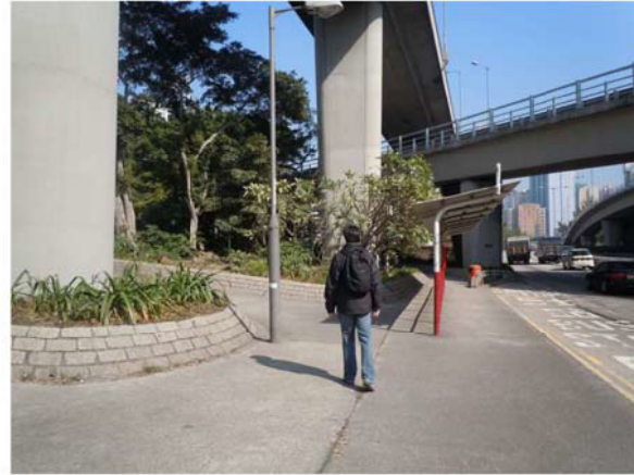
T2 Pedestrians travelling on Street Level under Kwai Chung Road Interchange Area
