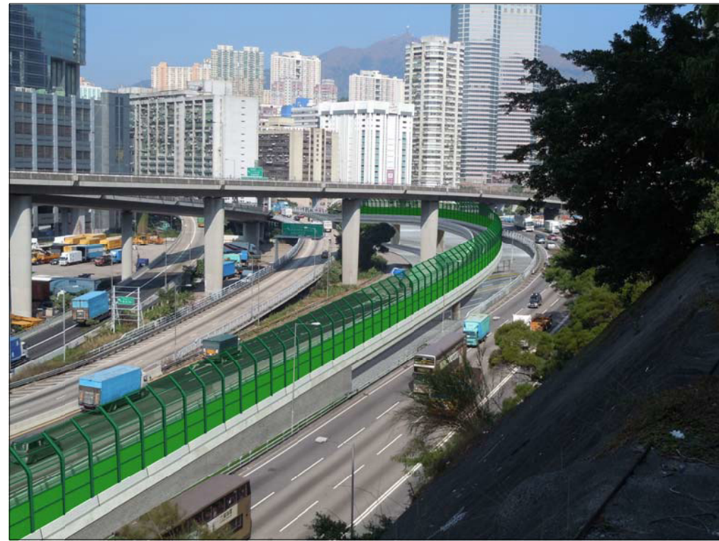
CASE 2 - PROPOSED FLYOVER FROM KWAI TSING INTERCHANGE UP-RAMP TO KWAI CHUNG ROAD
