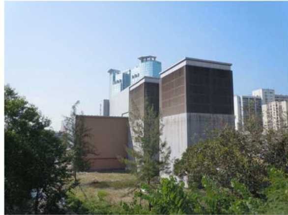
O3 Workers at Kwai Fong Ancillary Building
