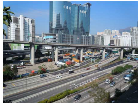
LCA6 Kwai Chung Road Interchange
