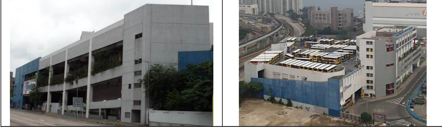
ASR 12: EMSD Depot
