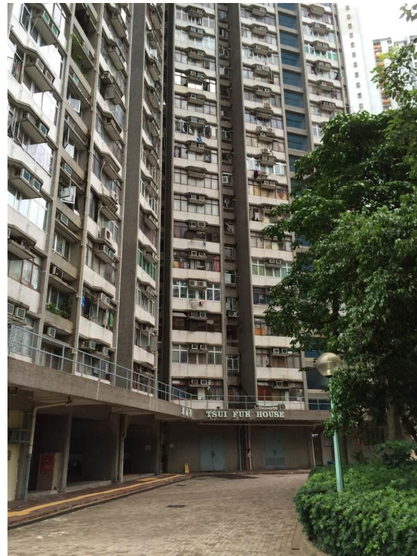
NSR 6 Tsui Fuk House, Tsui Wan Estate
