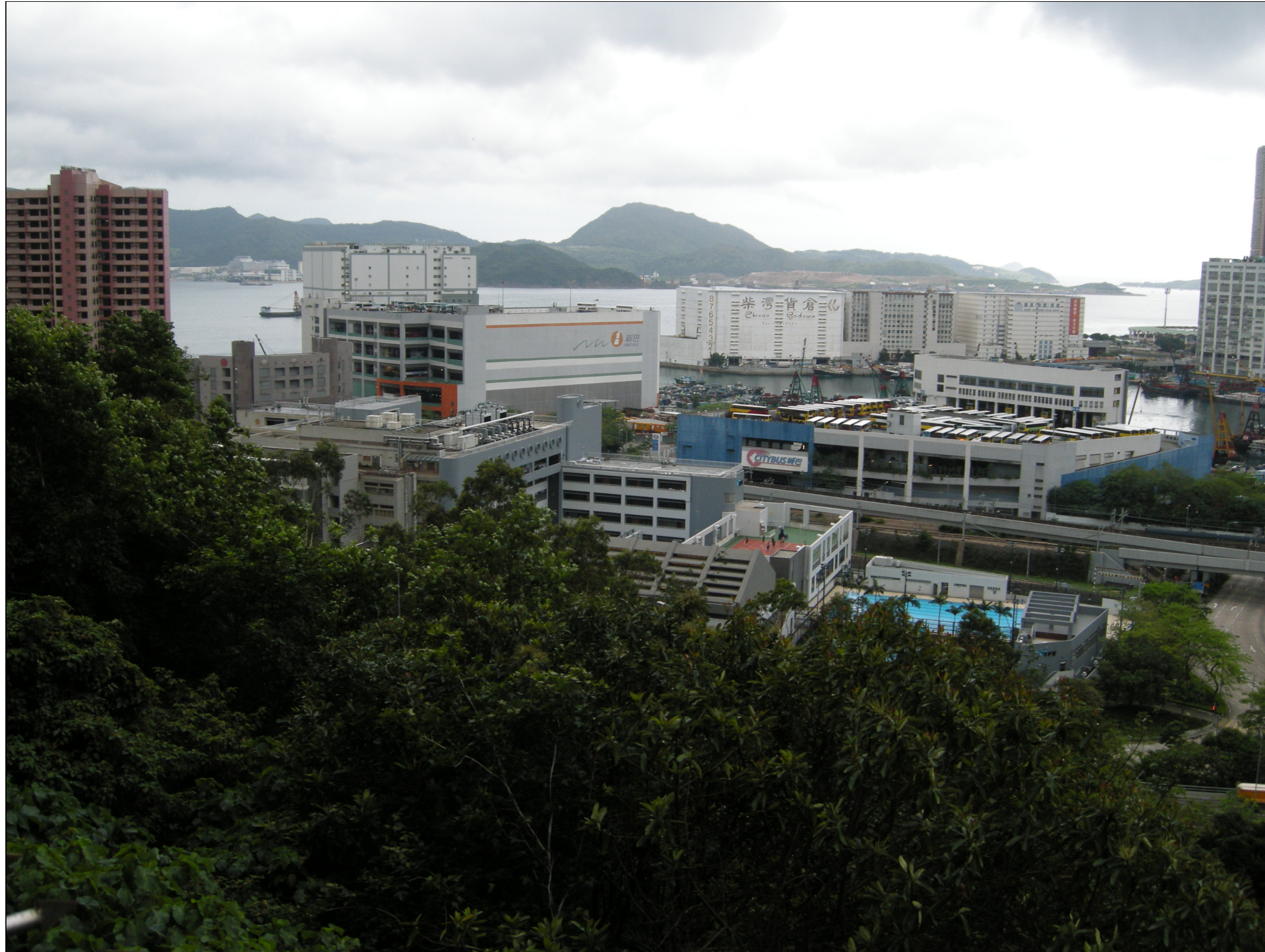
VP1: Block E of Pamela Youde Nethersole Eastern Hospital Senior Civil Servants Quarters Existing Condition
