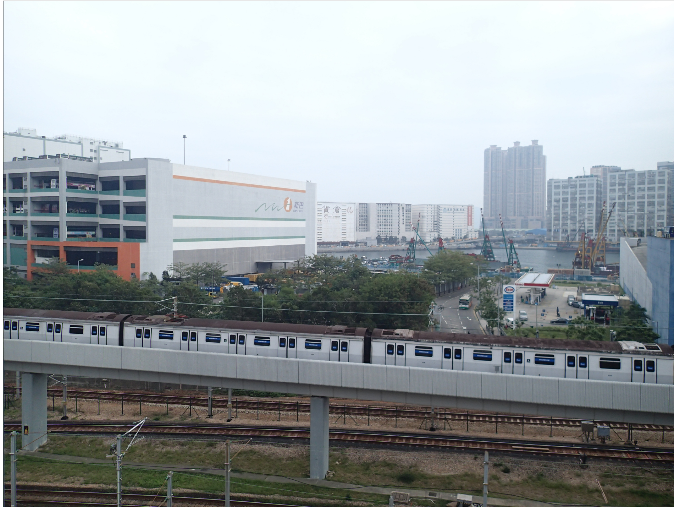
VP2: Hong Kong Institute of Vocational Education (Chai Wan) Existing Condition
