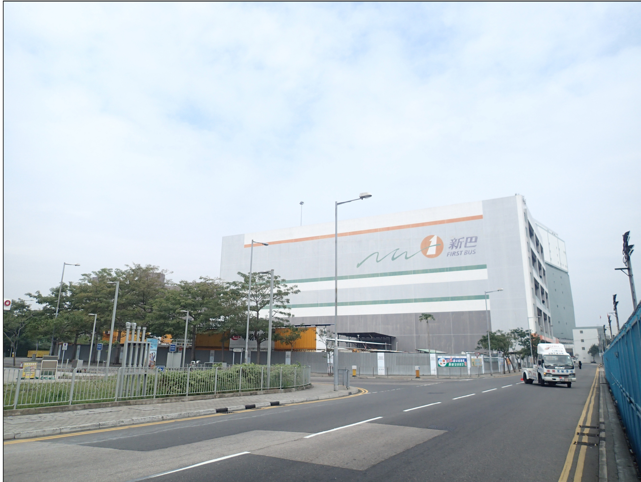
VP4: Sheung On Street Existing Condition
