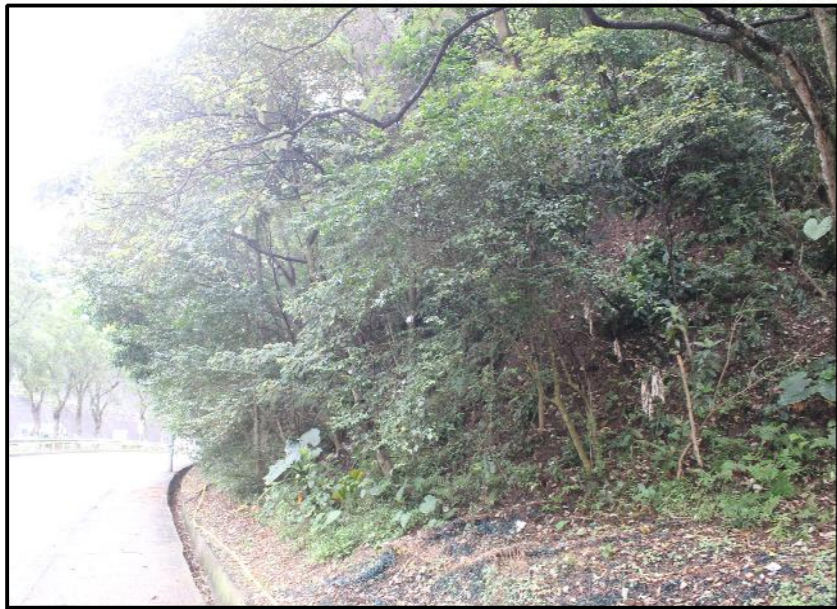
LR3.1 ENGINEERED SLOPE ALONG WITH SEMI-NATURAL DENSE HILLSIDE VEGETATION
