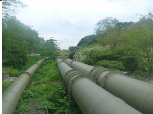
Plate 6 – View of the water pipes looking west to the south of the assessment area
