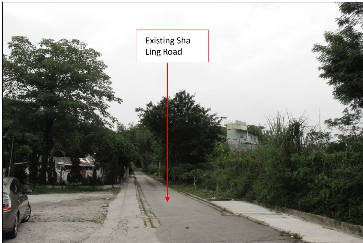
FROM VP1 EXISTING CONDITION
