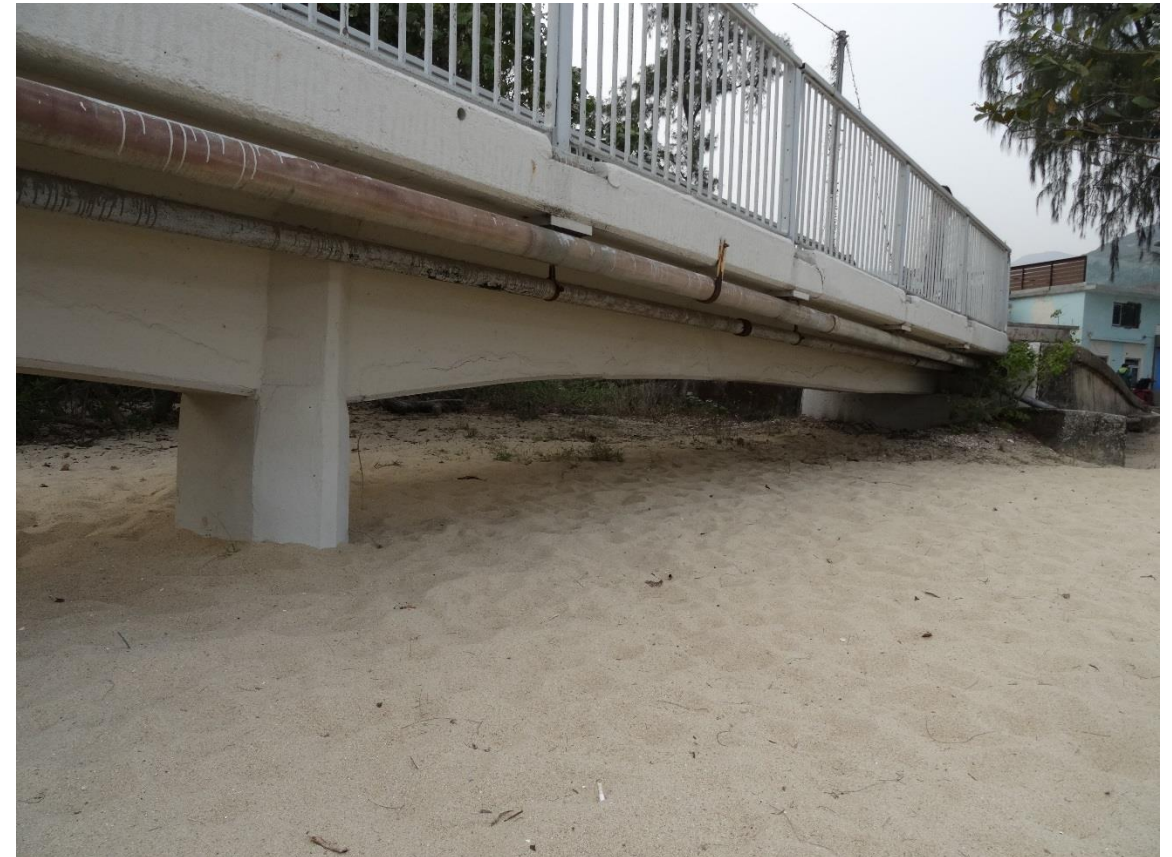
P2: Northern pier of Wang Tong Bridge
