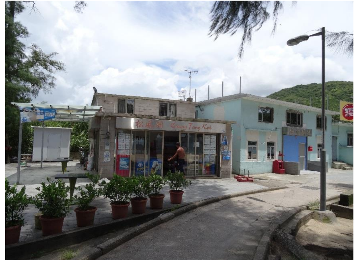
P6: Village House to the north of Wang Tong Bridge
