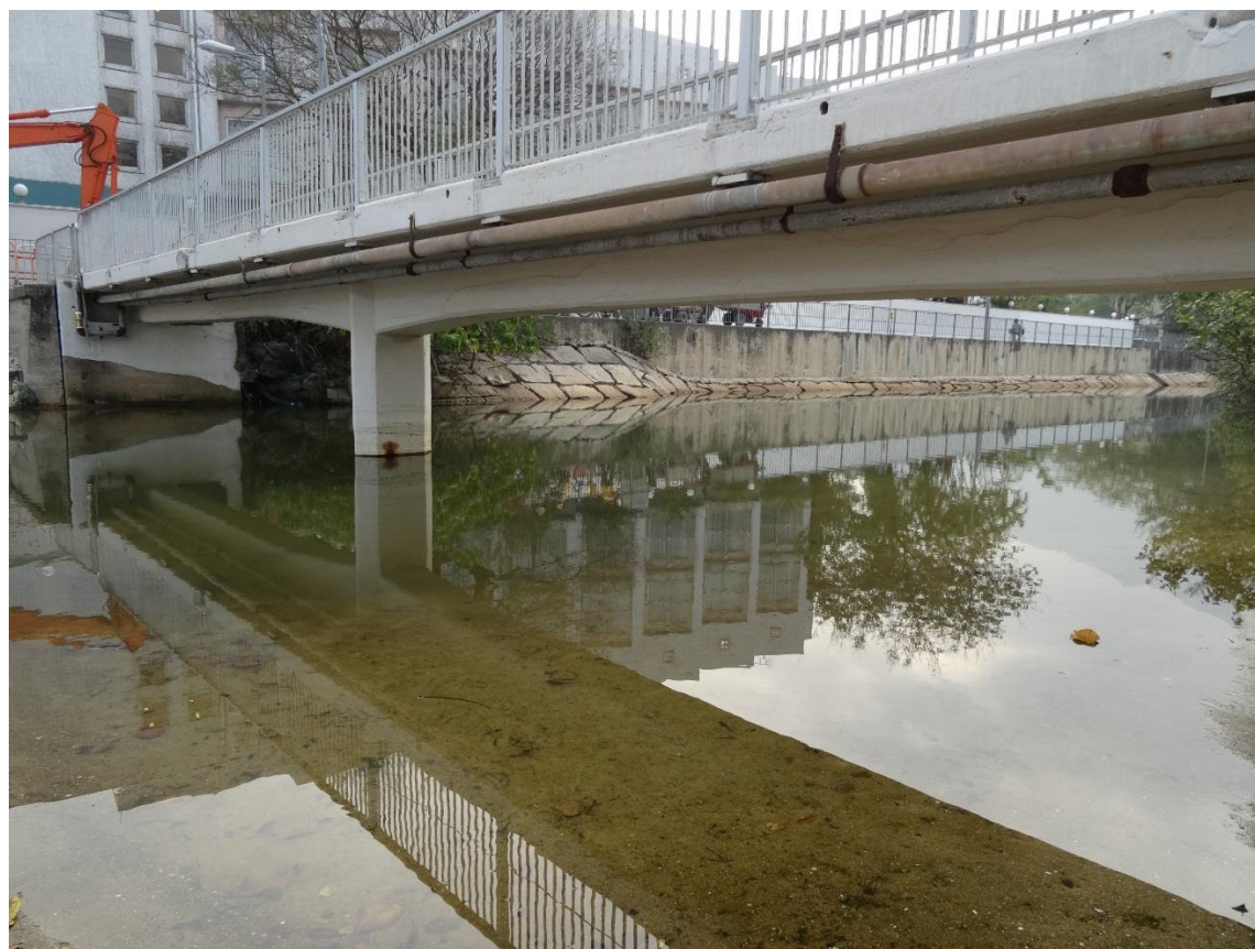
P3: Southern pier of Wang Tong Bridge
