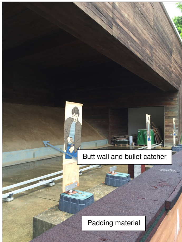
Figure 11-7: Padding material to prevent bouncing back of ricochet
