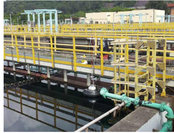
F9 - Final Sedimentation Tank
