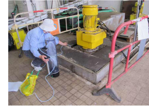
A4 - Digested Sludge Holding Tank
