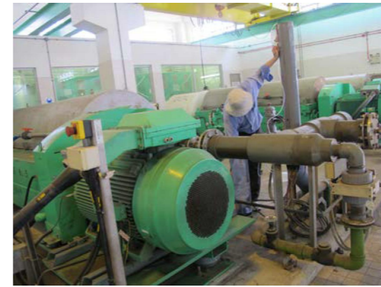
A3 - Thickened SAS Holding Tank
