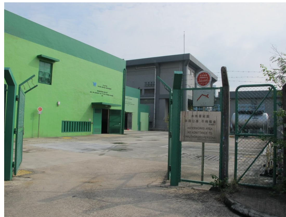
Figure 3 Sha Tin Seafront Salt Water Pumping Station
