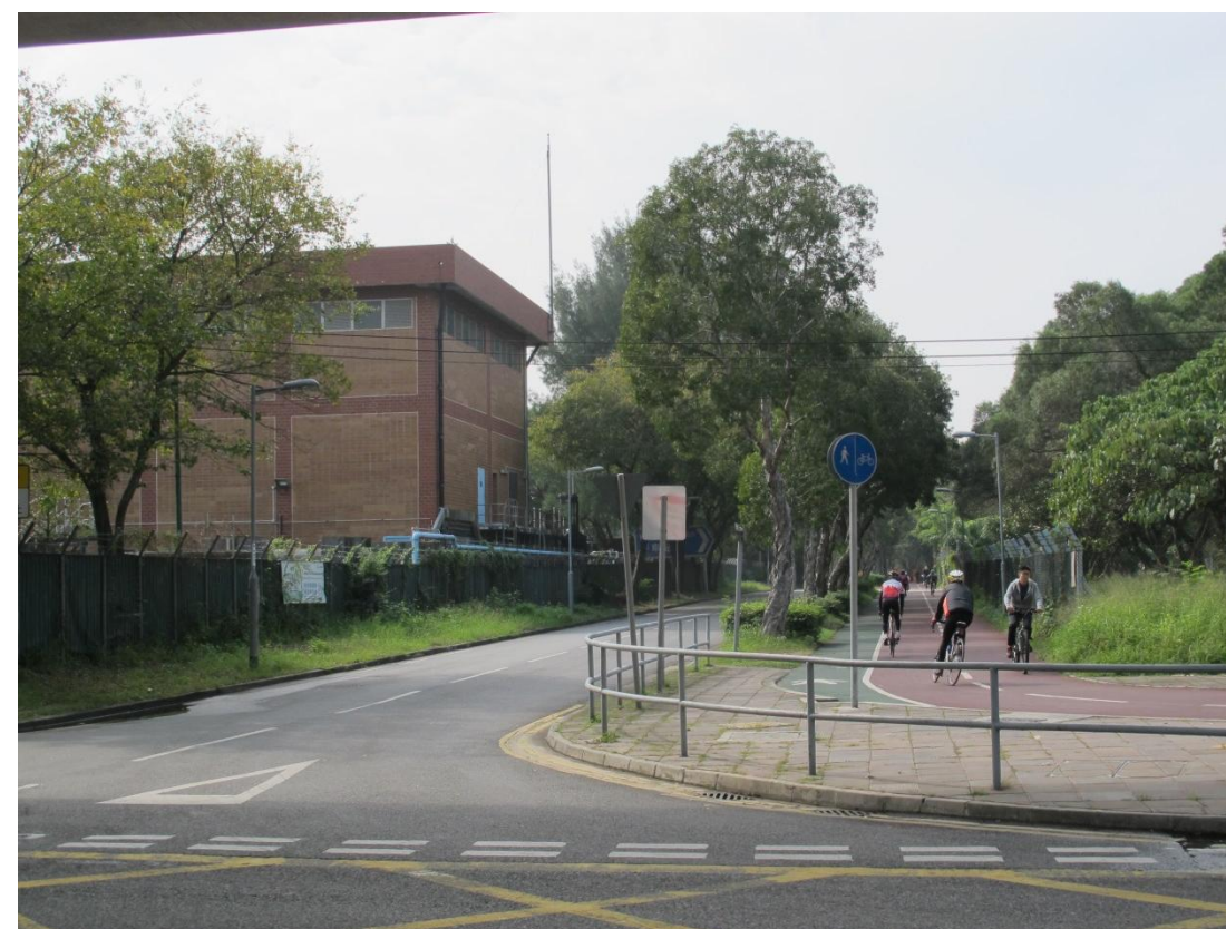
Figure 4 Effluent Pumping Station at Sha Tin Sewage Treatment Works
