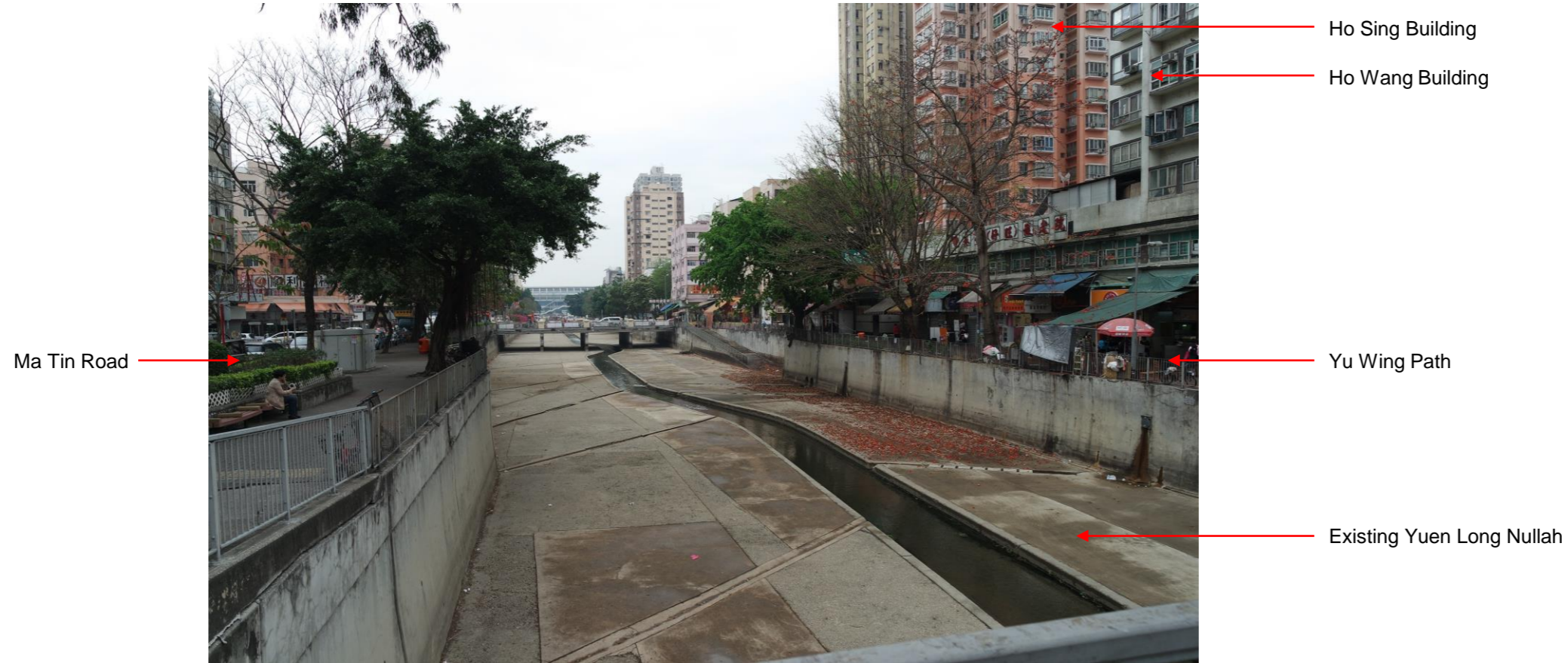
View REC9 – Existing Condition
