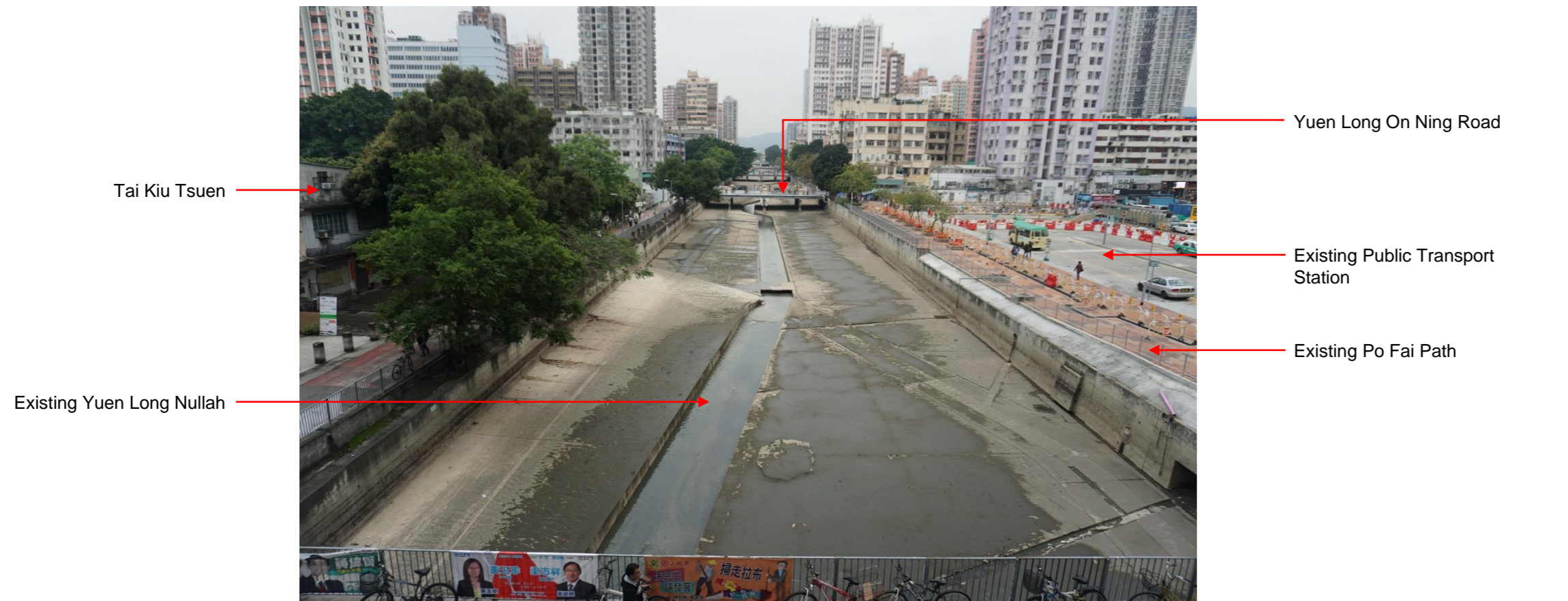
View REC1 – Existing Condition
