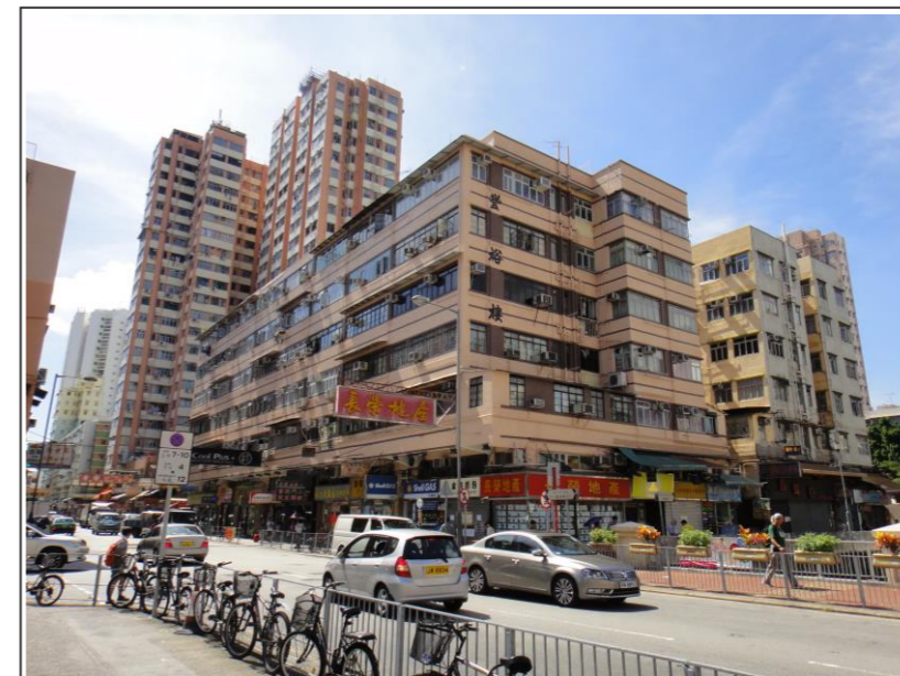
R3 - Kei Yip Building, On Ning Building, King Wah Building and Yuen Cheong House
