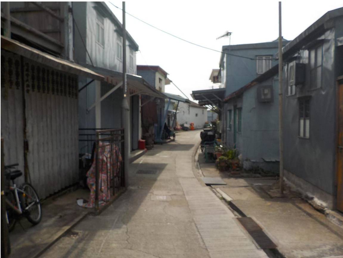
Photo 26 – Low-rise Residential Building at Shek Tsai Po Street
