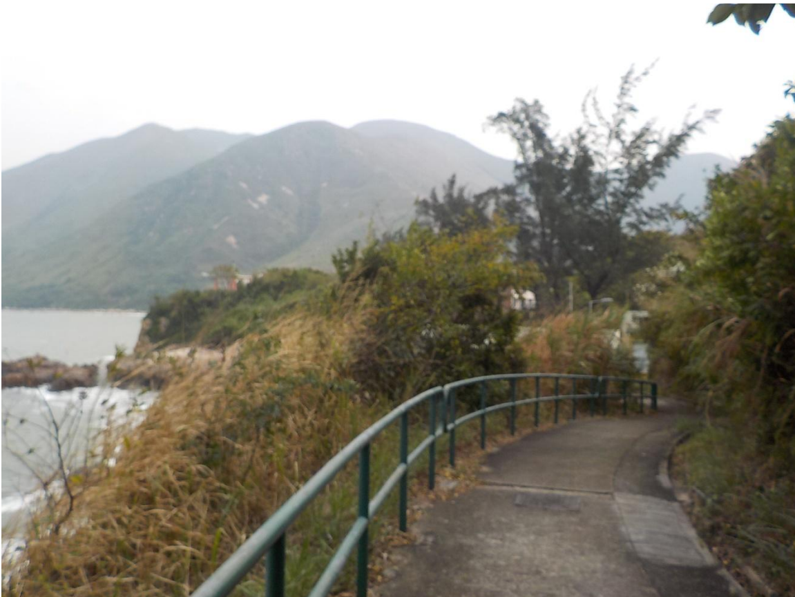
Photo 4 – Road leading to Existing STW
