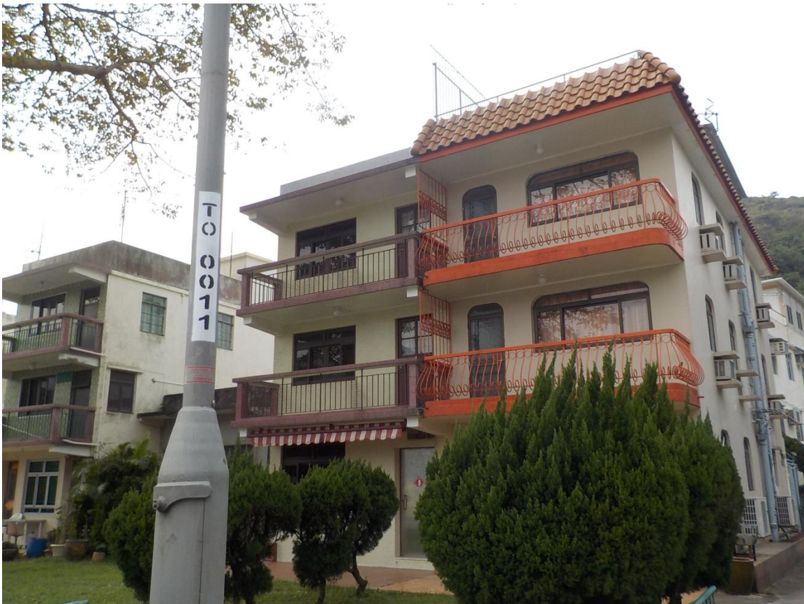
Photo 24 – Low-rise Residential Building at Shek Tsai Po Street
