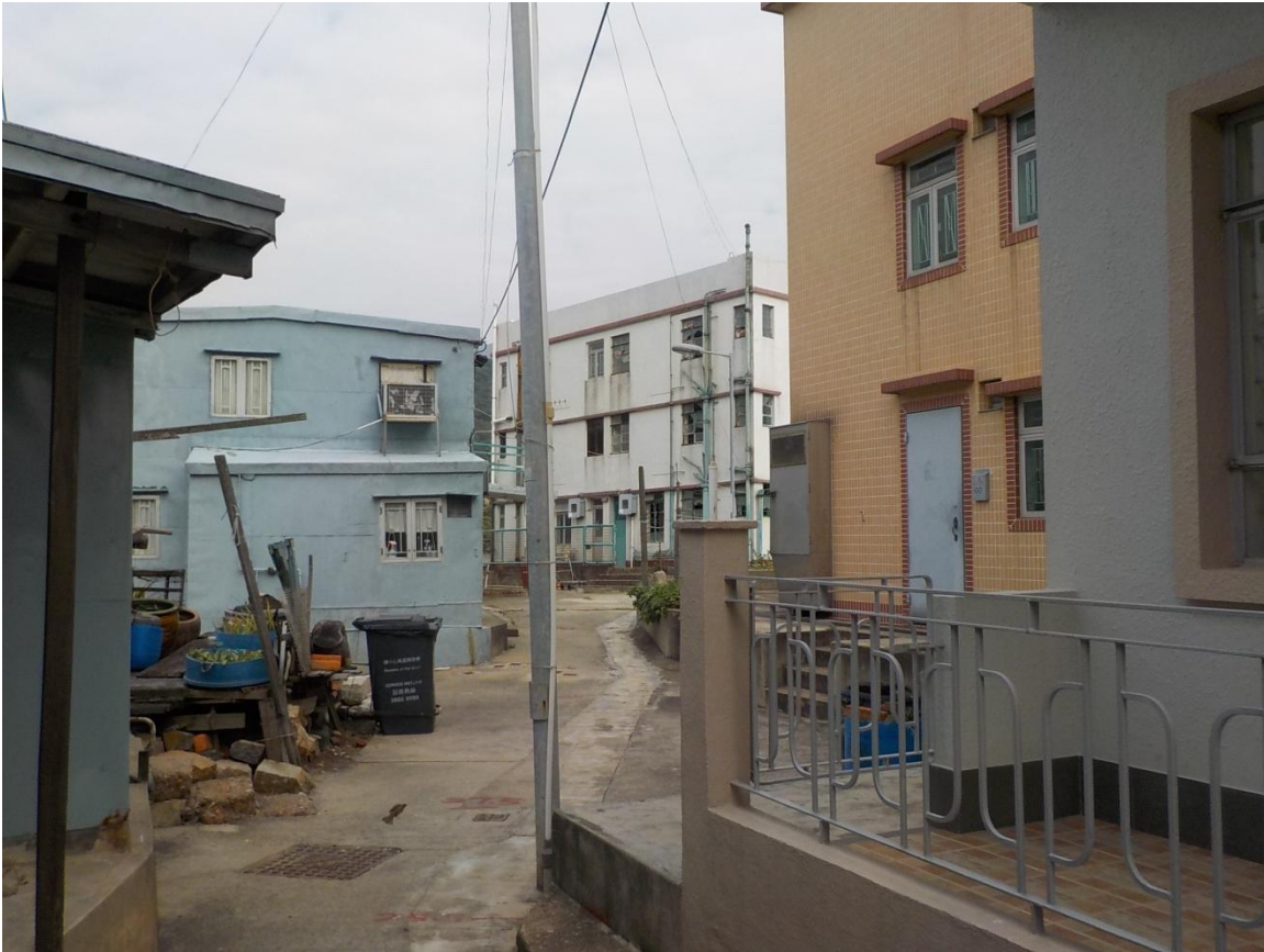
Photo 25 – Low-rise Residential Building at Shek Tsai Po Street
