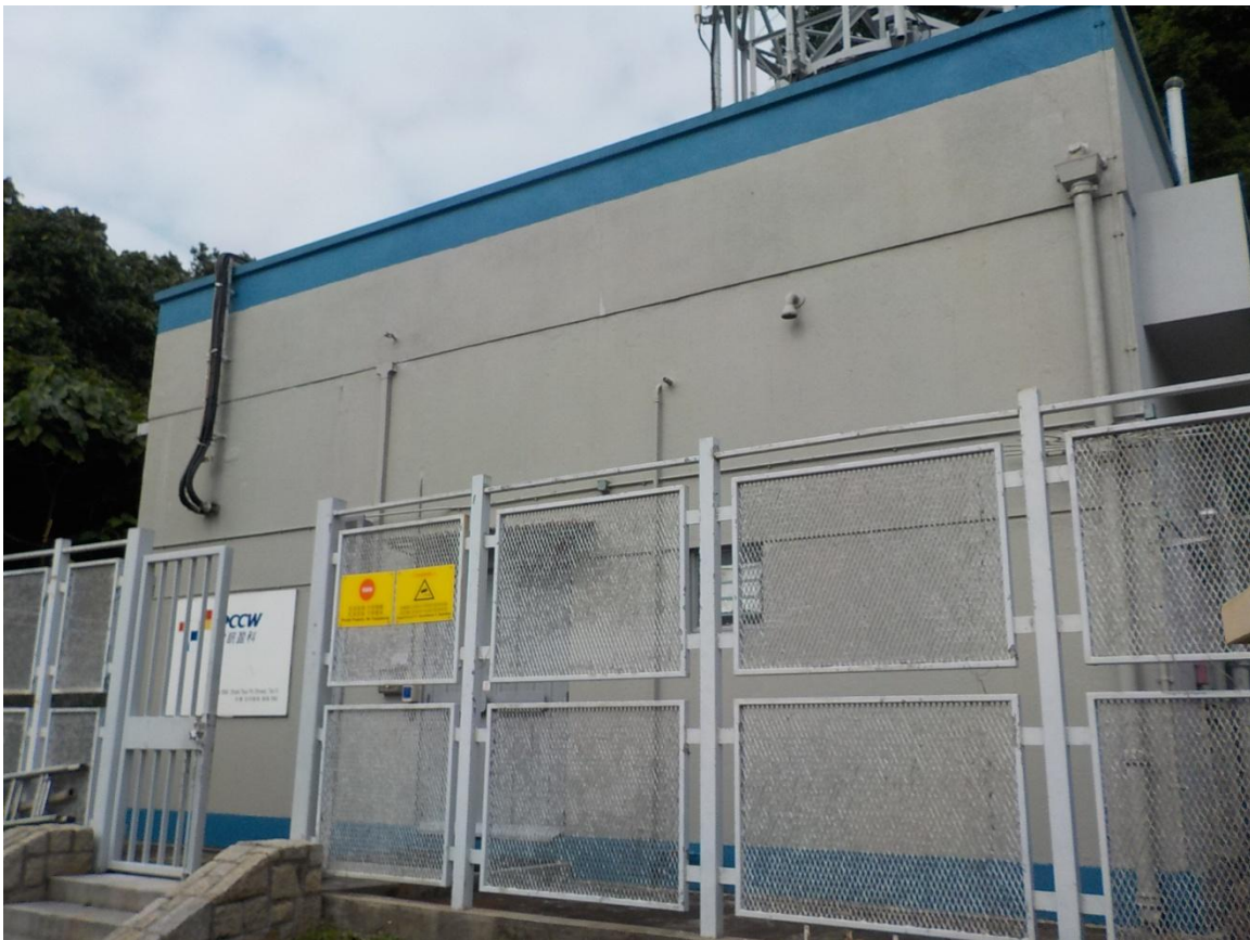
Photo 18 – Tai O Tel Exchange (CWP 5)
