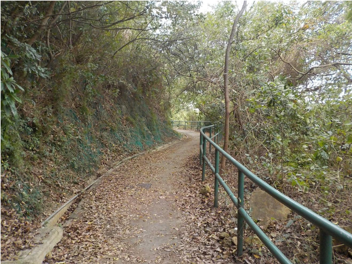
Photo 1 – Road leading to Existing STW
