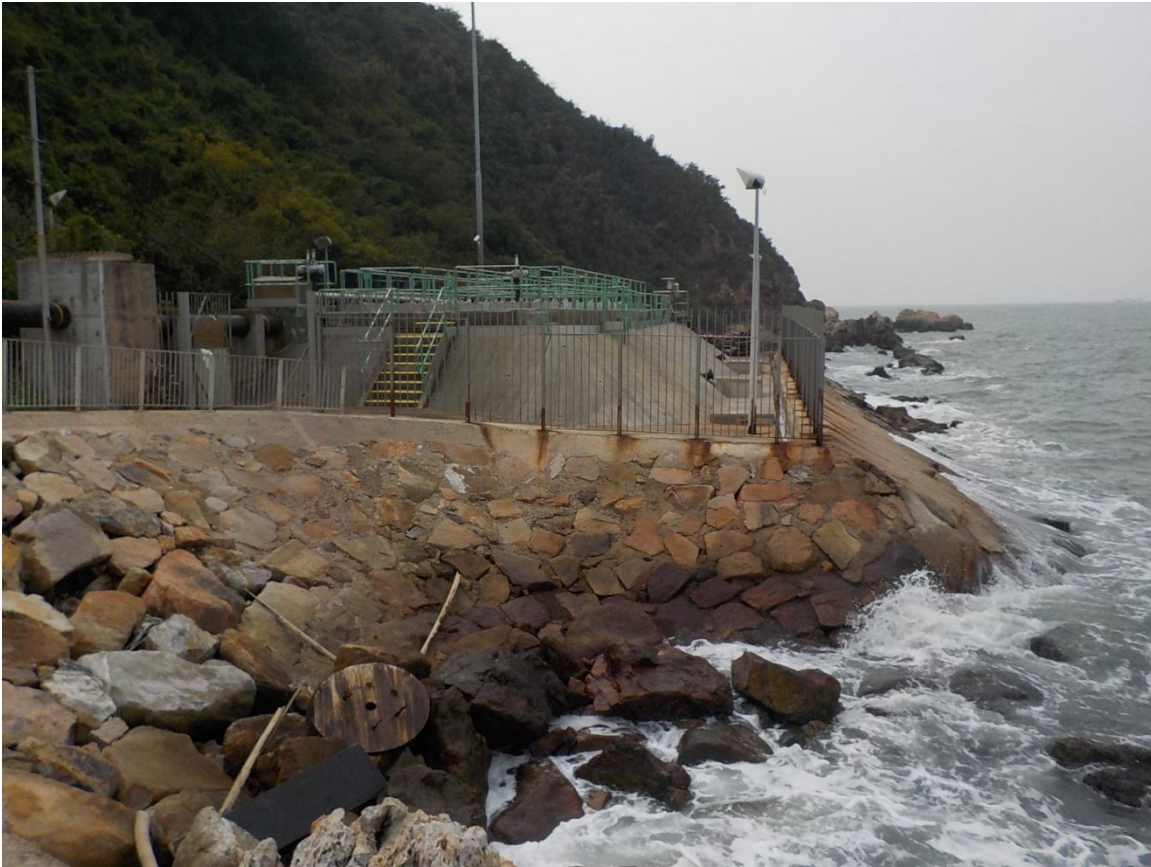
Photo 3 – View of Existing STW and Rising Main
