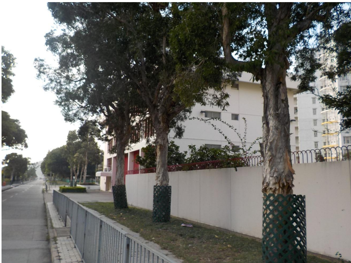
Photo 40 – Tai O Fire Station (at Tai O Road) (CWP 6)
